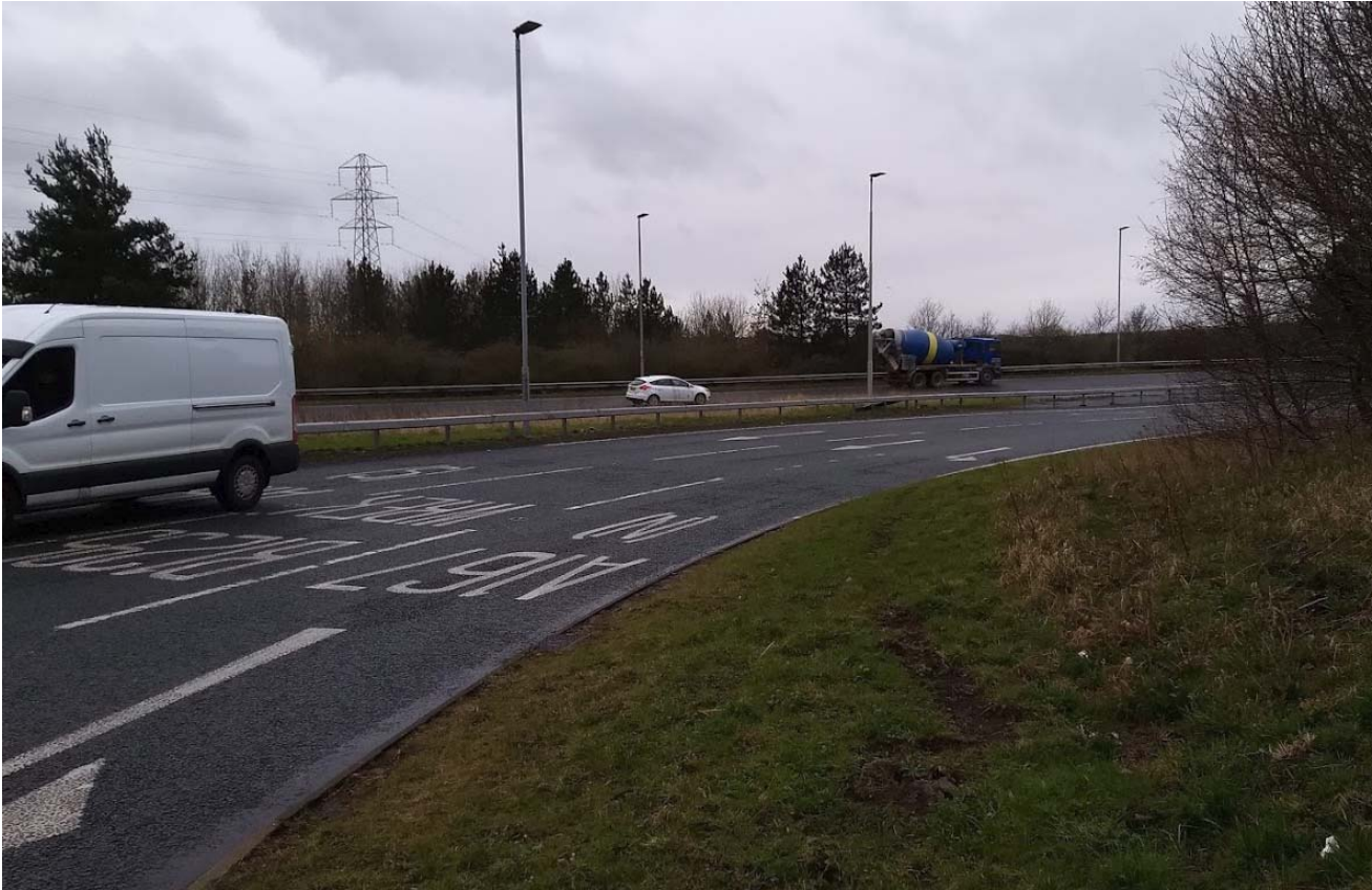
Figure 4-6 - Camber on the on/off slip
