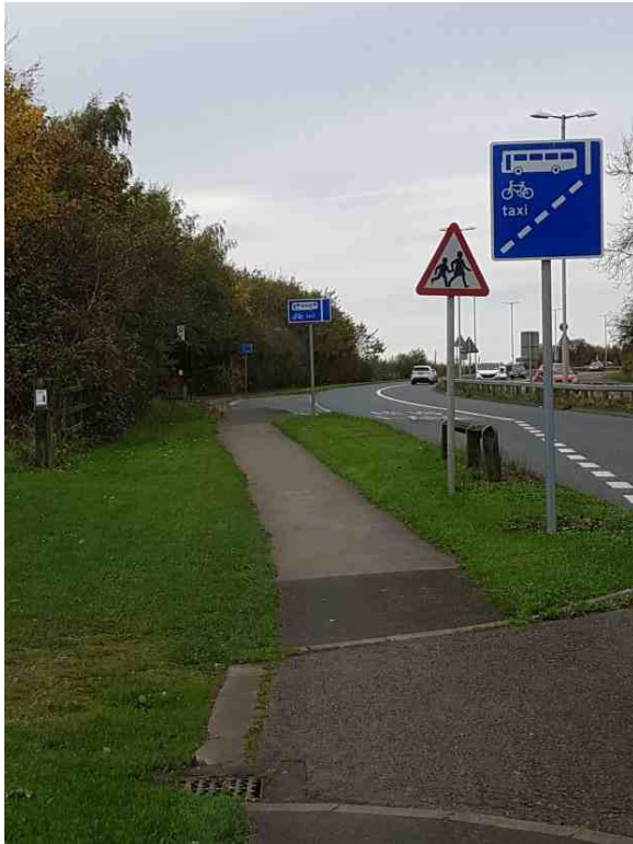
F.19 – Shared Footway/Cycleway provision taking facing north on the A167 Durham Road
