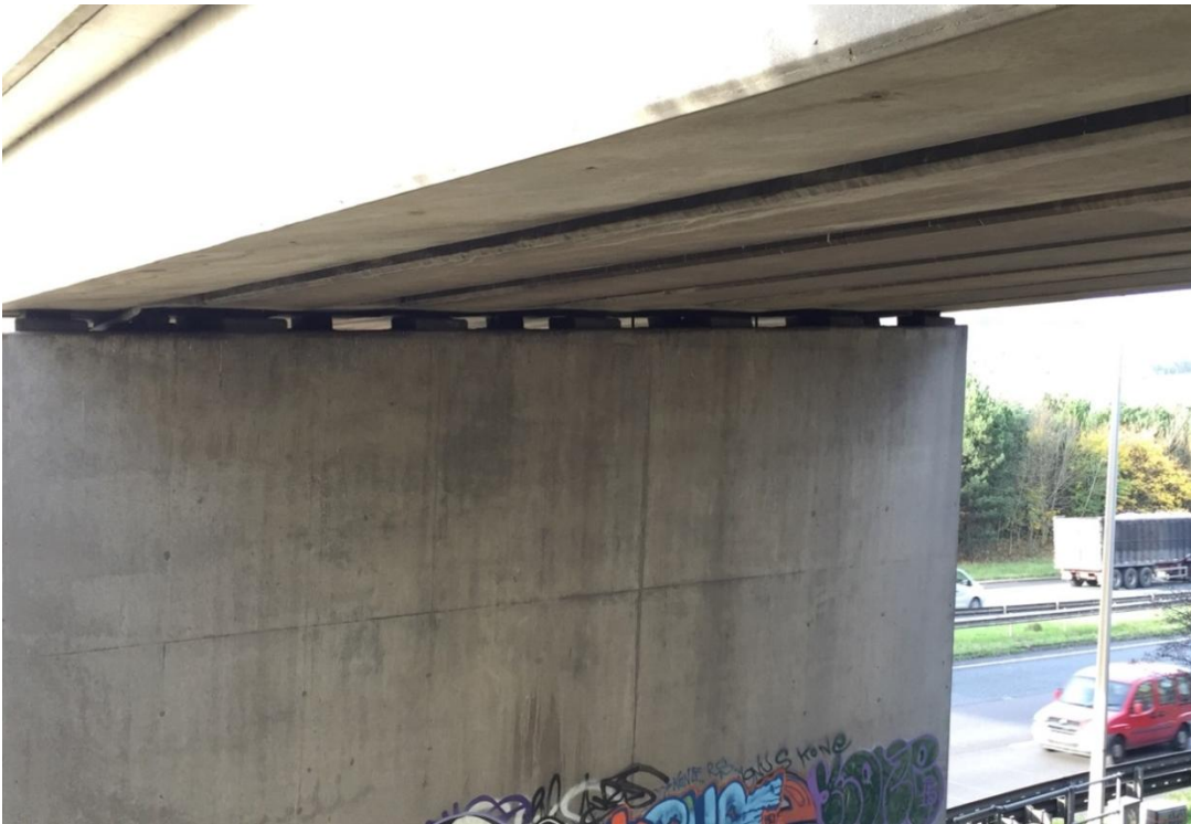
Photo 2- Potential roosting feature of the gaps between abutments and bridge deck on Smithy Lane Overbridge, as well as the gaps between the concrete beams on the underside of the bridge deck
