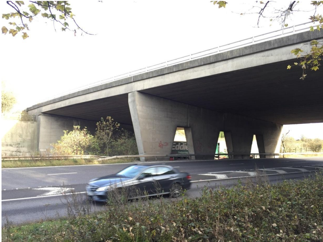
Photo 13- Lay out of North Side Overbridge
