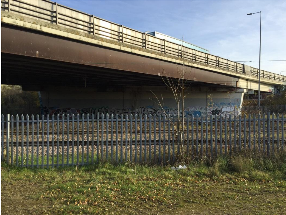
Photo 3- Layout of Allerdene Railway Underbridge
