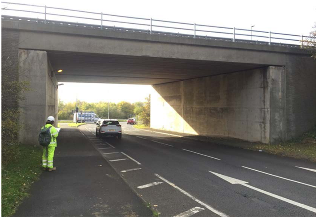
Photo 9- Layout of Eighton Lodge South Underbridge
