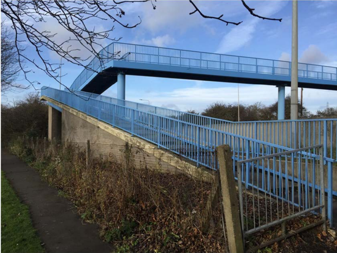
Photo 11- Lay out of North Dene Footbridge
