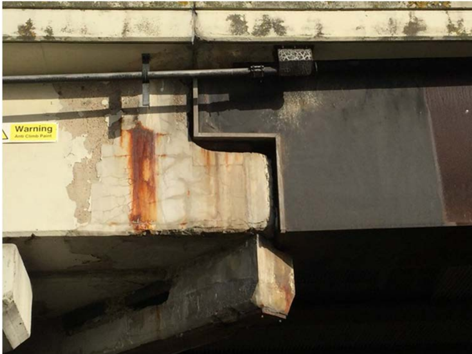
Photo 4- Potential roosting feature of the cavity between the concrete and steel deck structure on the southern end of the western pillar on Allerdene Railway Underbridge
