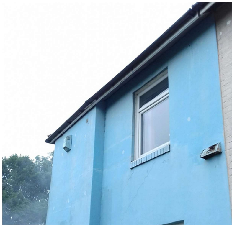
Photo 14 – North facing elevation of Building B2
