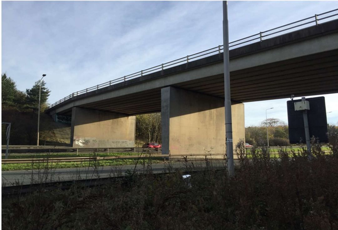
Photo 1- Layout of Smithy Lane Overbridge
