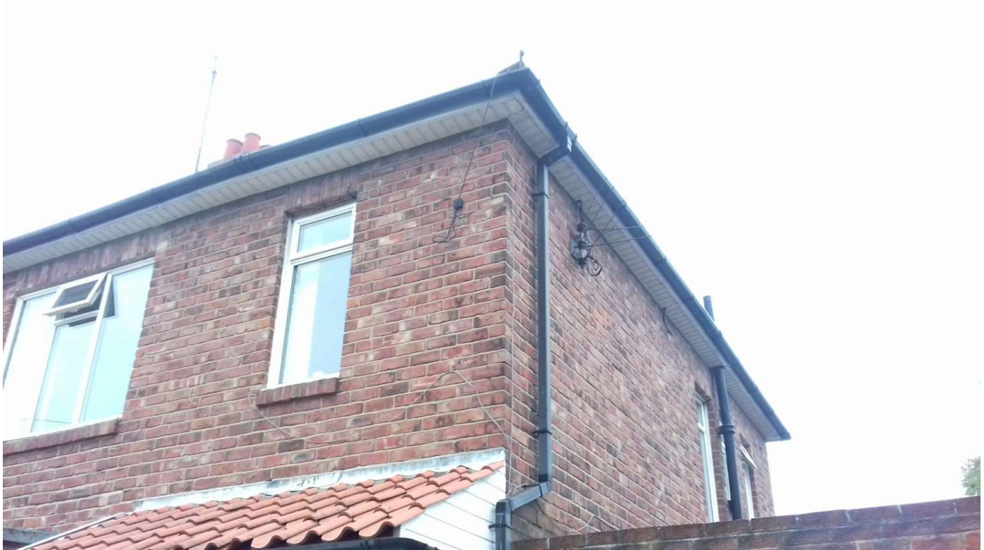
Photo 17 – North-west gable end of Building B1
