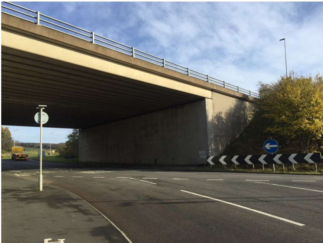
Photo 6- Layout of Eighton Lodge north underbridge
