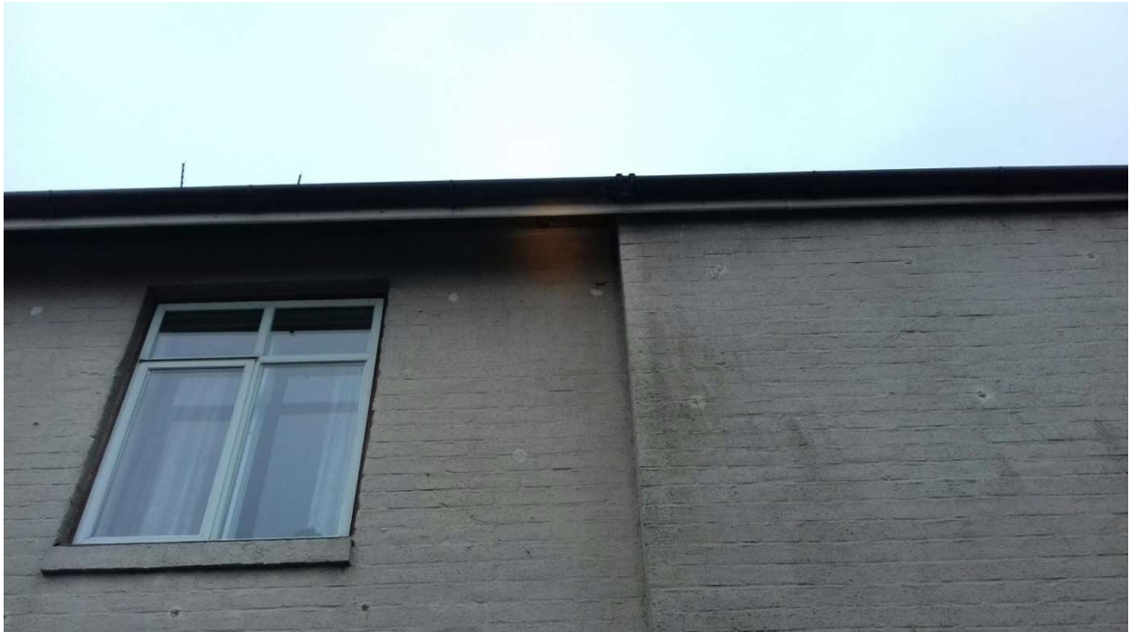
Photo 15 – North facing elevation of Building B2
