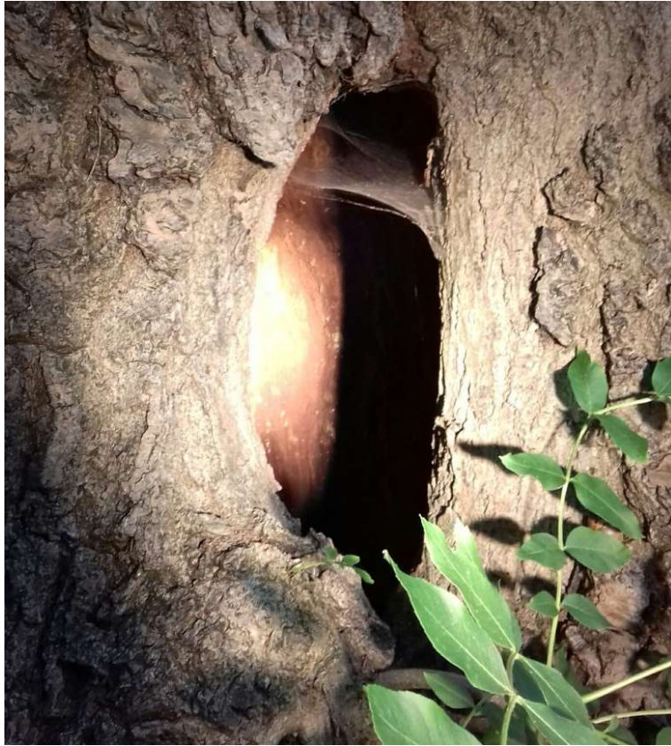
Photo 21 – A very advanced knot holes that has formed a large chest height rot hole in Tree T4
