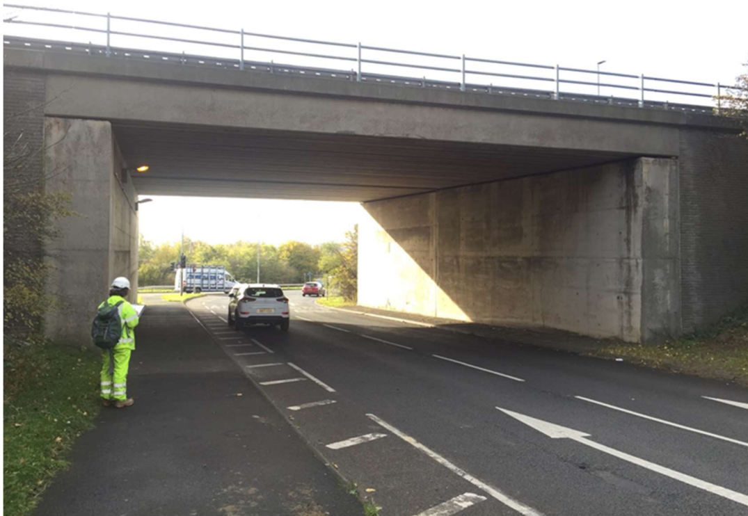
Photo 9- Layout of Eighton Lodge south underbridge
