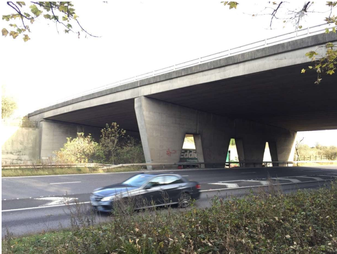
Photo 13- Lay out of Northside Overbridge
