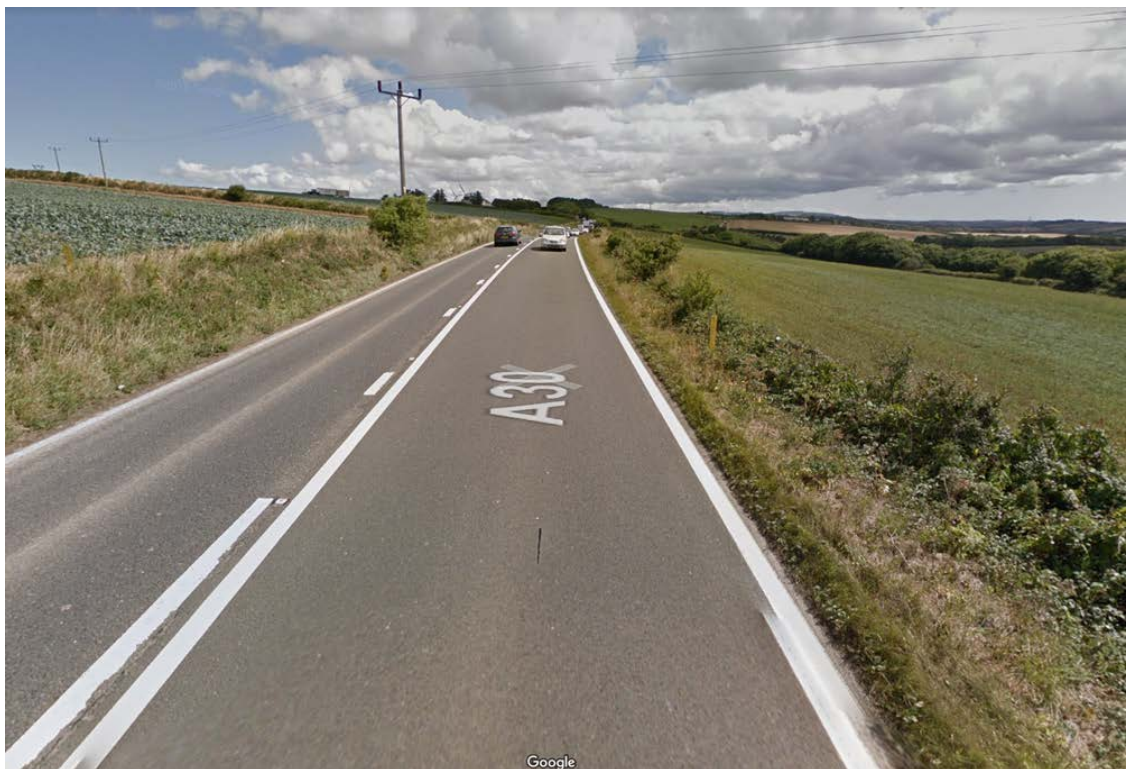
Figure 3.13 – Ennis Farm Junction to Raceland House
