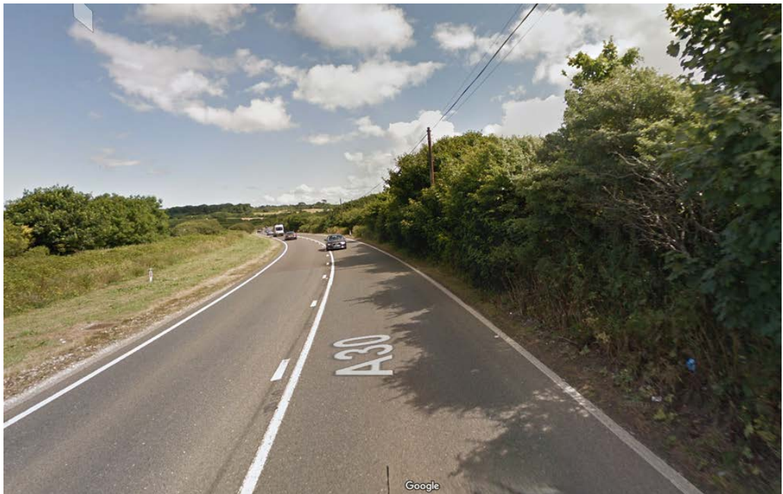
Figure 3.7 – Town & Country Access to Zelah bypass climbing lane Photo 1
