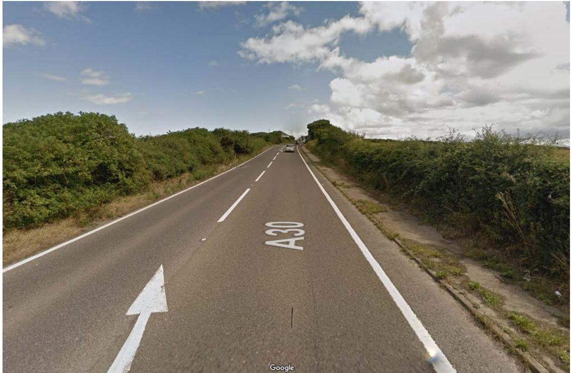
Figure 3.11 – Herver Lane junction to Boxheater Junction
