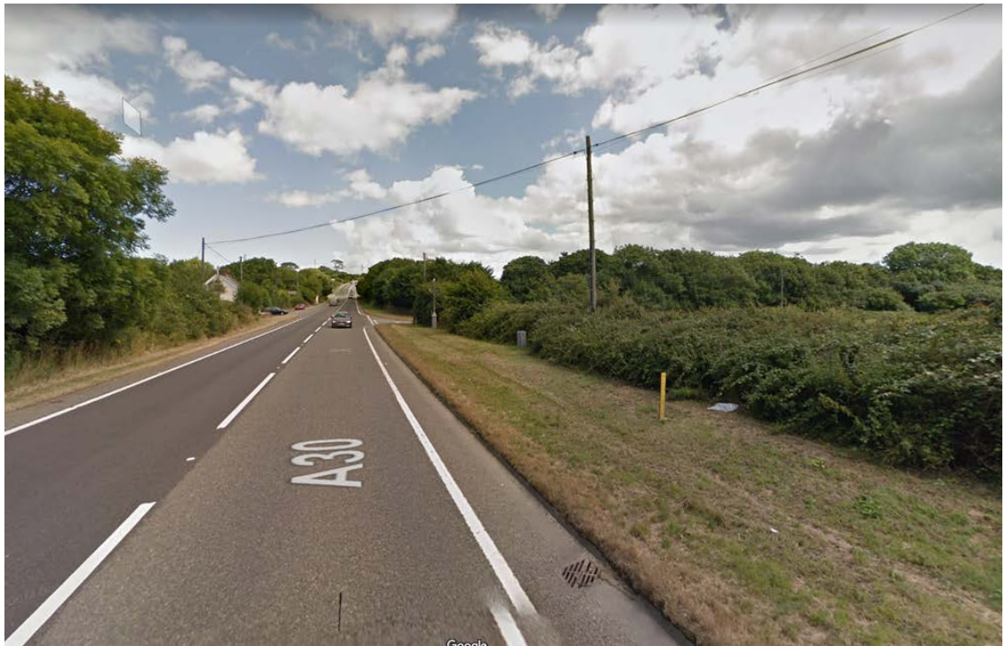
Figure 3.8 – Town & Country Access to Zelah bypass climbing lane Photo 2
