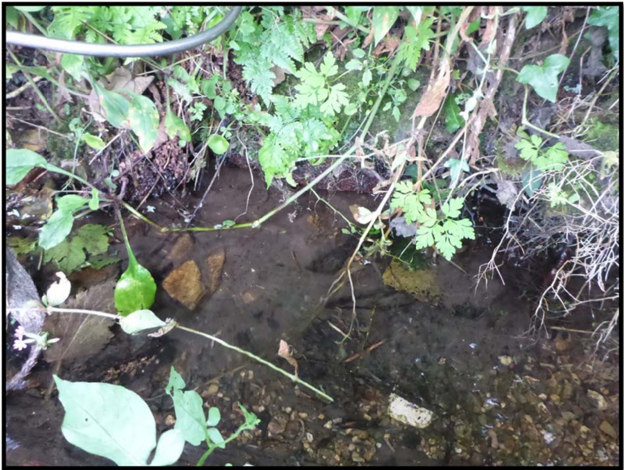
Figure 14 Sediment ingress in marginal areas at Site 13.4
