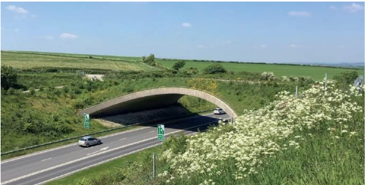
Figure 8: General example of a green bridge, as proposed for Land Bridge 4. (Source: A303 Amesbury to Berwick Down TR010025 Environmental Statement Non-Technical Summary Volume 6.0 APFP Regulation 5(2)(a) Planning Act 2008 Infrastructure Planning (Applications: Prescribed Forms and Procedure) Regulations 2009 October 2018, page 6).
