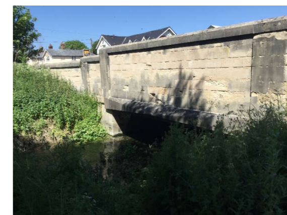
Photo IMG_0086: A303 road bridge
