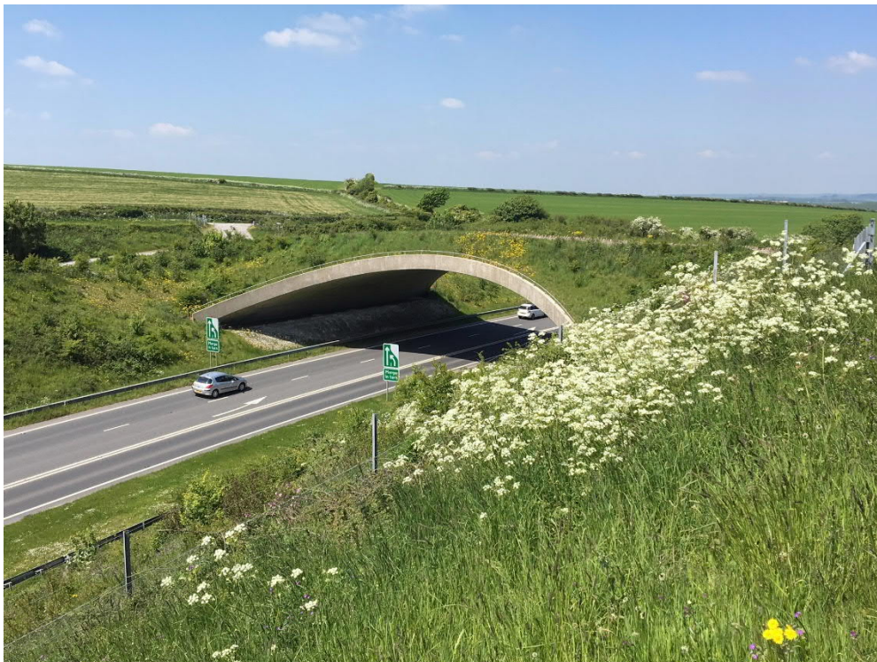
Figure 2.3: Example of a green bridge (Weymouth Relief Road)
