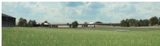
Option 1: Open parapet which would make the viaduct less visually intrusive but would mean high-sided vehicles would be more visible and there would be less noise screening
