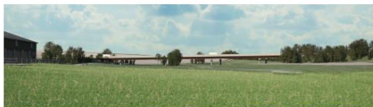
Option 2: Parapet screen would maintain the continuity of the visual and noise screening provided by proposed landscaped banks either side of the viaduct
