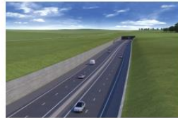
Approach option with vertical retaining walls
