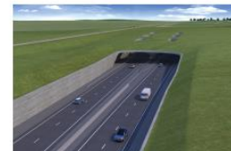
Grassed over canopy with ventilation outlets
