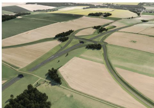
View of the new Longbarrow junction looking south west
