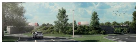
Option 1: Two single-span bridges over the existing roundabout, with the centre filled in with landscaped slopes
