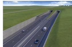
Western tunnel entrance - vertical retaining walls option
