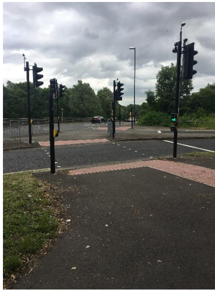
23: Signal controlled crossing on the bridge over the A38. RCR 66
