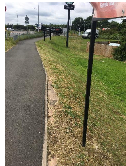
6: NCN 54 looking South with steep embankment
