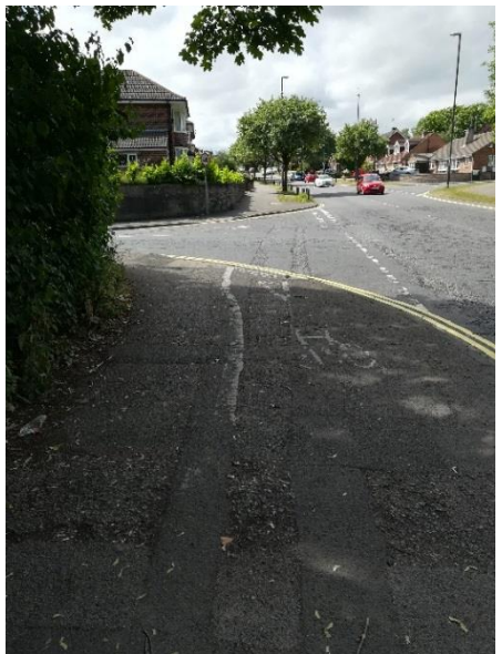
36: Brackensdale Avenue junction with Greenwich Drive South
