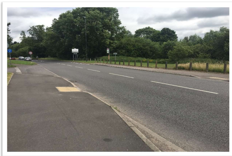
Figure 3: Uncontrolled crossing point, Alfreton Road
