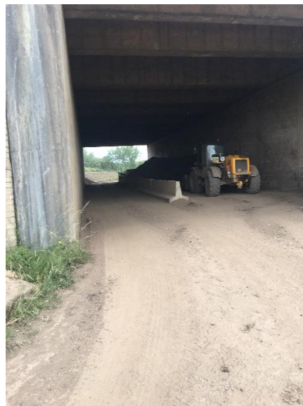
17: Existing underpass under A38 following Breadsall footpath 7
