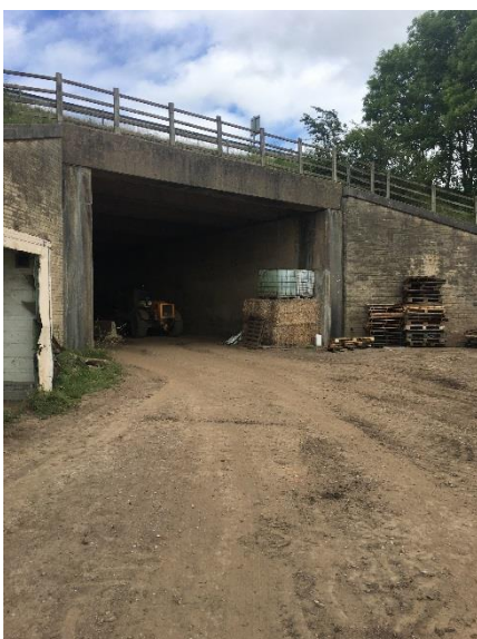
16: Existing underpass under A38 following Breadsall footpath 7
