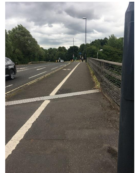
24: RCR 66 Follows Kedleston Road over A38
