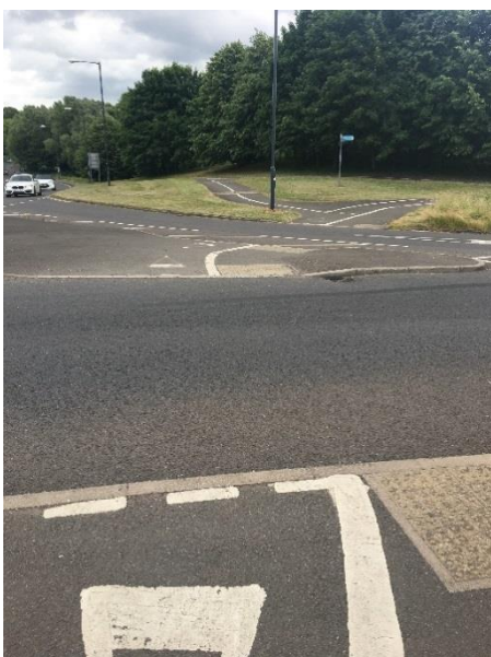
25: RCR 66 Un-controlled crossing across A38 entry slip
