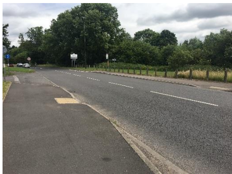
4: Un-controlled crossing point across B6179
