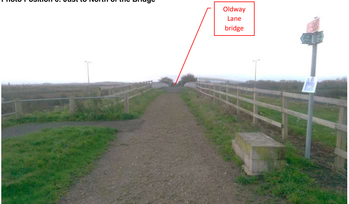
Looking South towards Oldway Lane bridge
