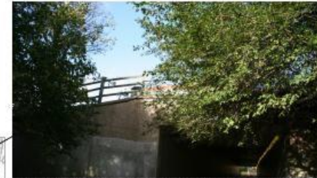
Fig 1.0: View from south of St Dunstan's underpass/ rear of stables
