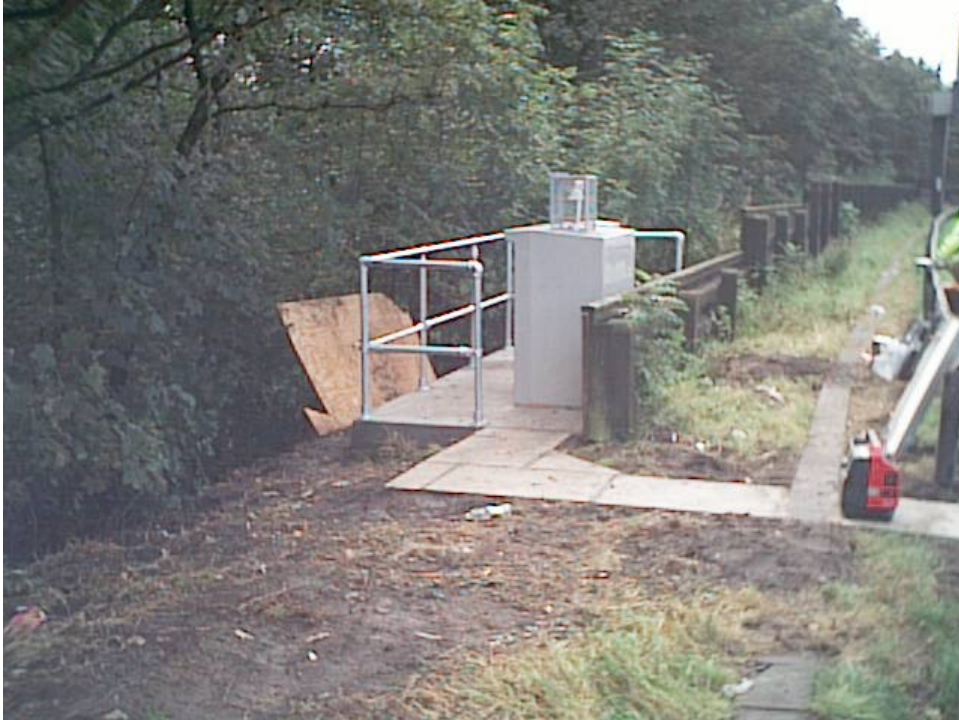
Figure 2.4 – Lower Northern End of Original Barrier
