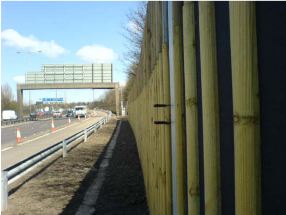
Figure 2.3 – Standard Barrier Section
