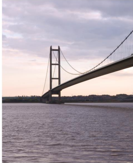
The project will bring opportunities to the Humber, safeguarding existing jobs and putting the region at the forefront of carbon capture technology in the UK.
