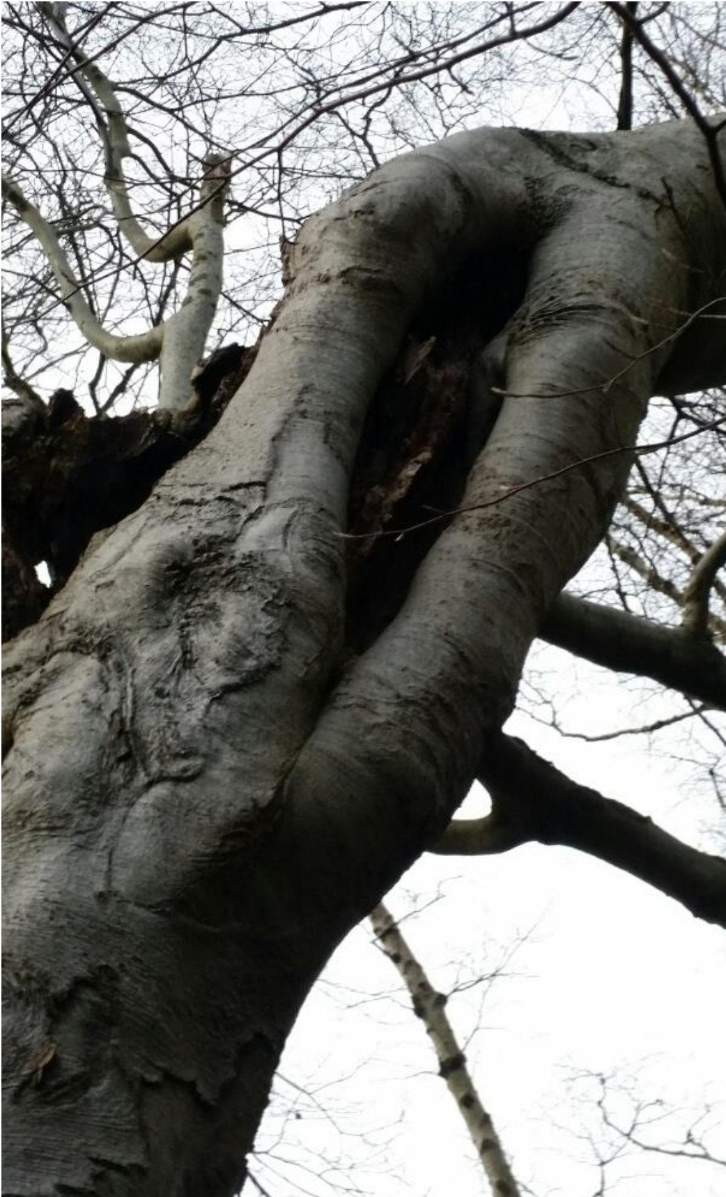
RBC-009 Cavity in main stem of beech with moderate roosting potential
