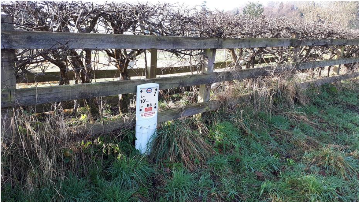
Photograph 4.2: Typical industry standard pipeline marker post
