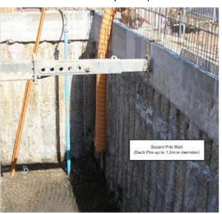
While this approach substantially reduces the rate of flow to the excavation, there will still be a residual groundwater abstraction to maintain dry and safe conditions within the structure.
