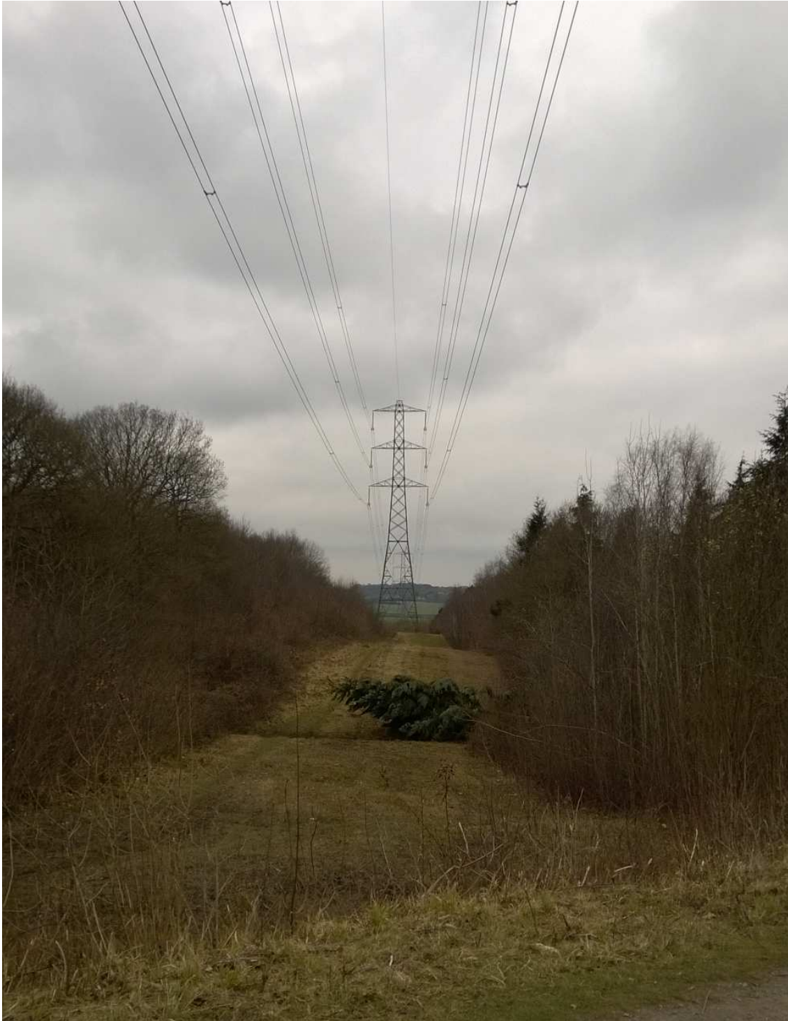
Fig 2: 400kV OHL passing through Clowes Wood looking north-west
