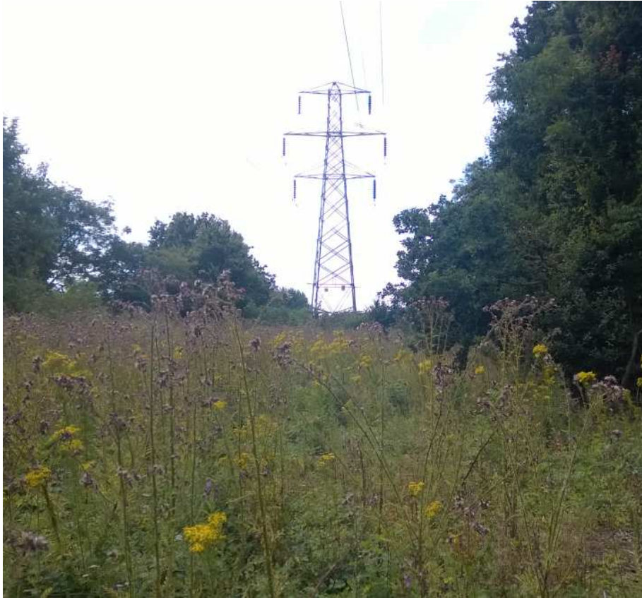
Fig 3: 132kV PX OHL passing through Dengrove Wood looking west
