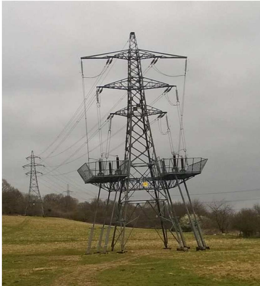
The image above shows a transition from OHL to underground cable at Folly Farm on the outskirts of Canterbury. This forms part of the PX 132kV line. The image below shows a transition on an EHV transmission line in the Netherlands. We accept that something larger in area may be required on the Richborough Connection, with security fencing and other safety features. However being at ground level these features can easily be screened by suitable planting.
