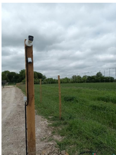
Image 3.5 – Example wire-mesh deer stock fencing and security camera
