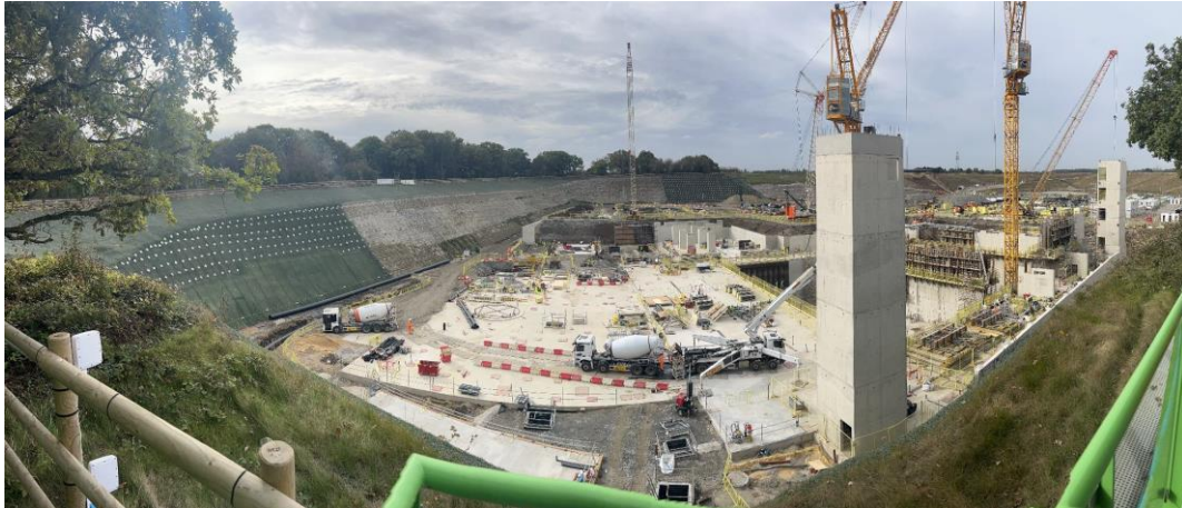
Figure 2: Existing Consent under Construction
