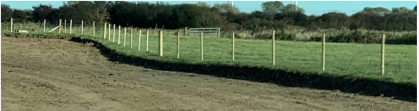
Figure 1.2: Example of post and wire fencing
