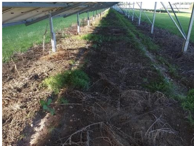
Welsh Government Report - Figure 6: Channels created by panel runoff within 12 months of site operation commencing
