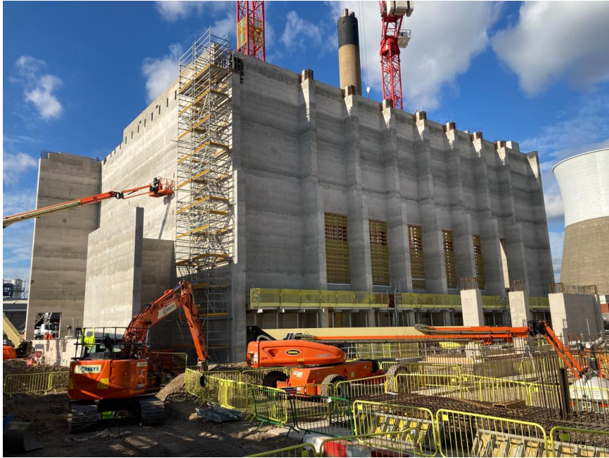
Plate 2.3 – Consented Scheme Tipping Hall slab supports under construction (Date: October 2021)
