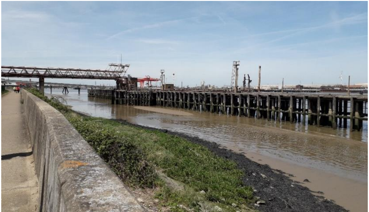
Figure 1-1: Belvedere Power Station Jetty - View from the Thames footpath
