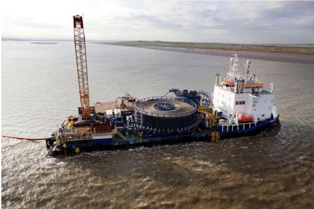
Graphic 4-13 Example export cable installation vessel (Rampion 1 offshore wind farm)
