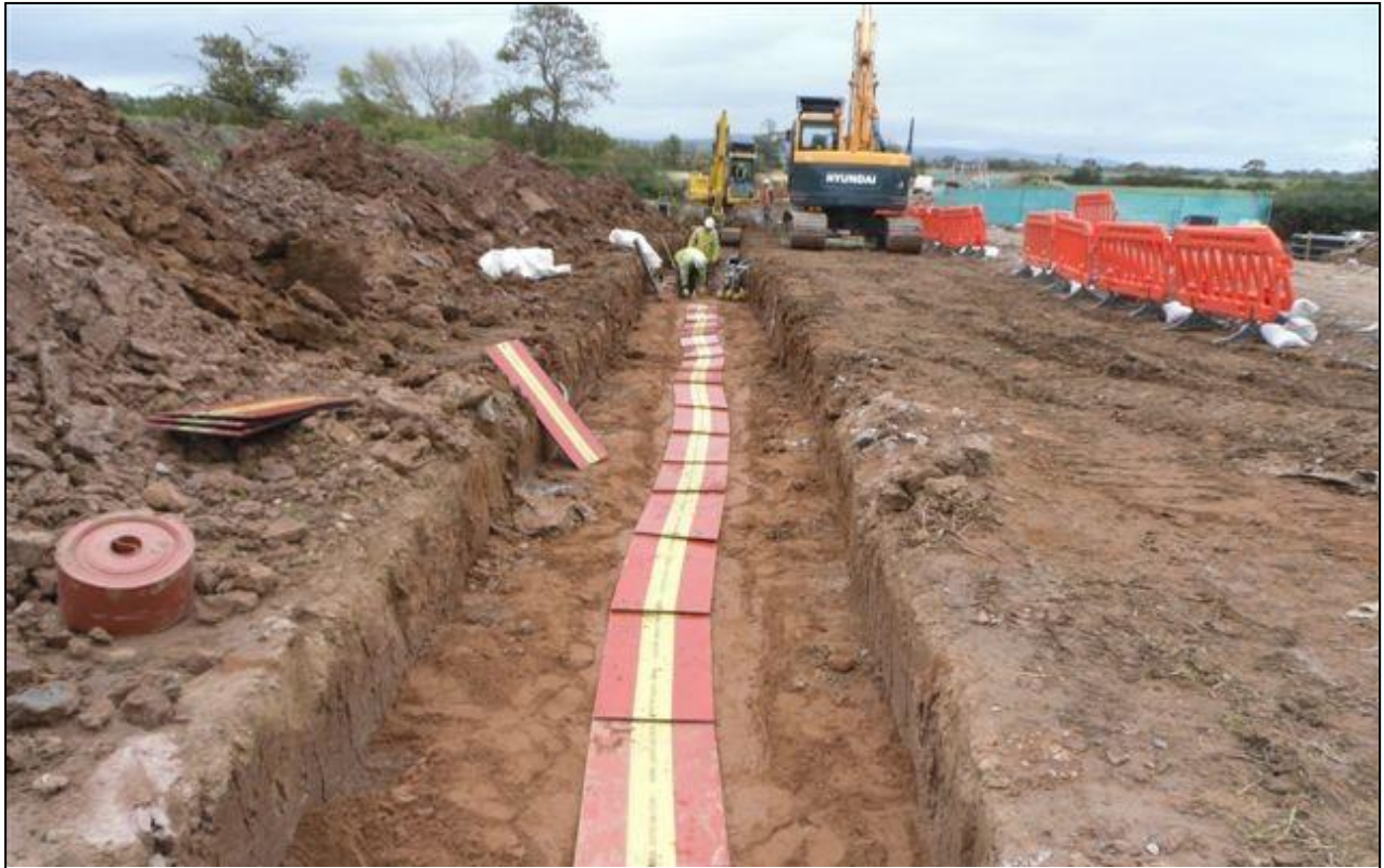
Figure 27: Cable trench having been partially backfilled, with cable marker boards (courtesy of RWE renewables UK Ltd).
