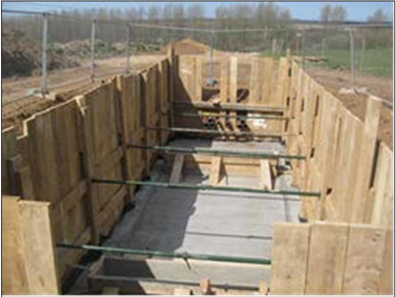
Figure 28: Typical joint pit under construction (courtesy of RWE renewables UK Ltd)
