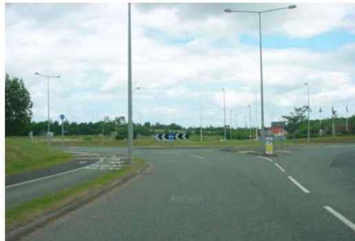
Picture 12. St Asaph Business Park roundabout at OS Grid Ref SJ 016 746. Load approaches from centre left of camera and turns right towards camera. Contraflow of this roundabout is recommended.
