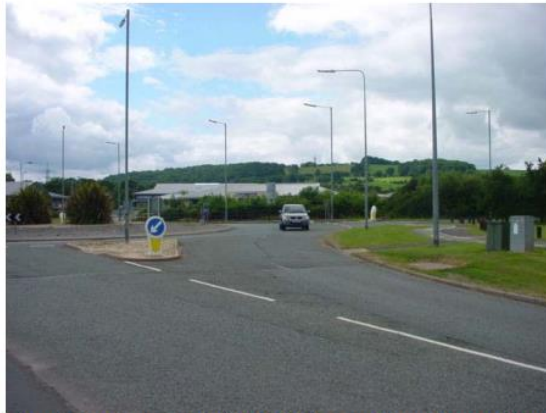
Picture 14. St Asaph Business Park/B5381 Glascoed Road roundabout. On route 3, loads turn right at this roundabout which for 20 axle frame trailers would be best undertaken in contraflow. Caution is required in relation to lamp posts and street furniture but the turn is considered negotiable.
