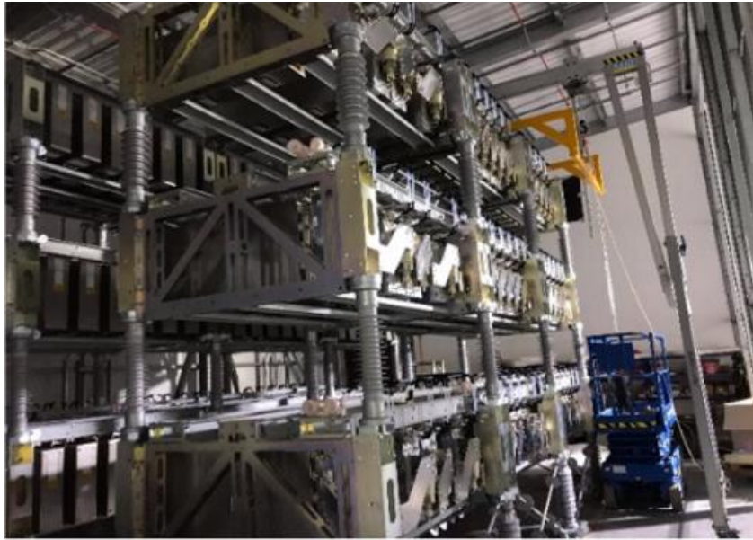
Figure 1: Example SVC solutions - Triton Knoll reactive compensator/SVC with the temporary crane beam in place during construction.
