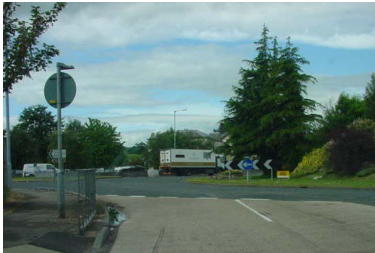
Picture 1. A55 westbound exit slip road onto A525. Load comes from behind camera and turns left.
