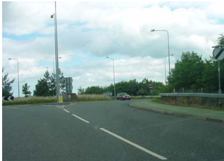
Picture 11. Exit from A55 to St Asaph Business Park. Load approaches from centre right of camera from A55 westbound exit slip road and turns left towards camera.
