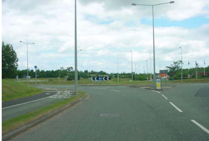
Picture 12. St Asaph Business Park roundabout at OS Grid Ref SJ 016 746. Load approaches from centre left of camera and turns right towards camera. Contraflow of this roundabout is recommended.
