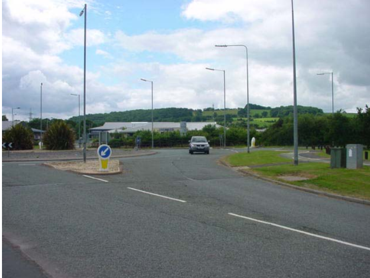
Picture 14. St Asaph Business Park/B5381 Glascoed Road roundabout. On route 3, loads turn right at this roundabout which for 20 axle frame trailers would be best undertaken in contraflow. Caution is required in relation to lamp posts and street furniture but the turn is considered negotiable.
