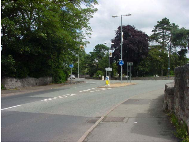
Picture 2. A525 The Roe /B5381 Glascoed Road roundabout. Load moves towards camera from top left of picture. Contraflow of the island may be necessary with removal of street furniture including lamppost, keep left sign and directional signs.
