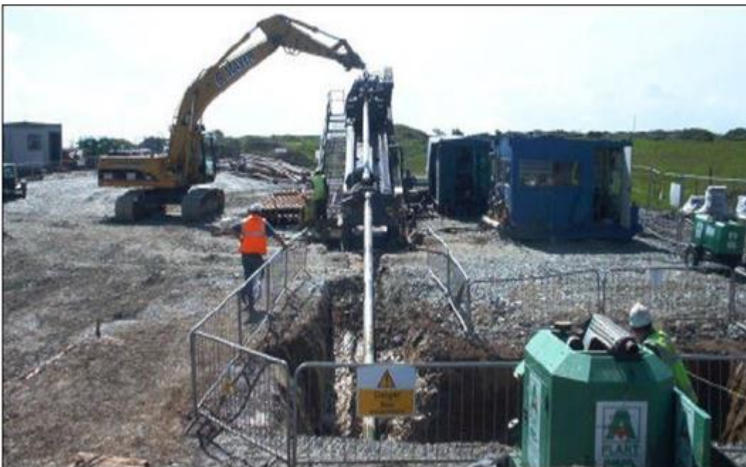
Figure 20: Illustrative visualisation of a landfall HDD Installation.
