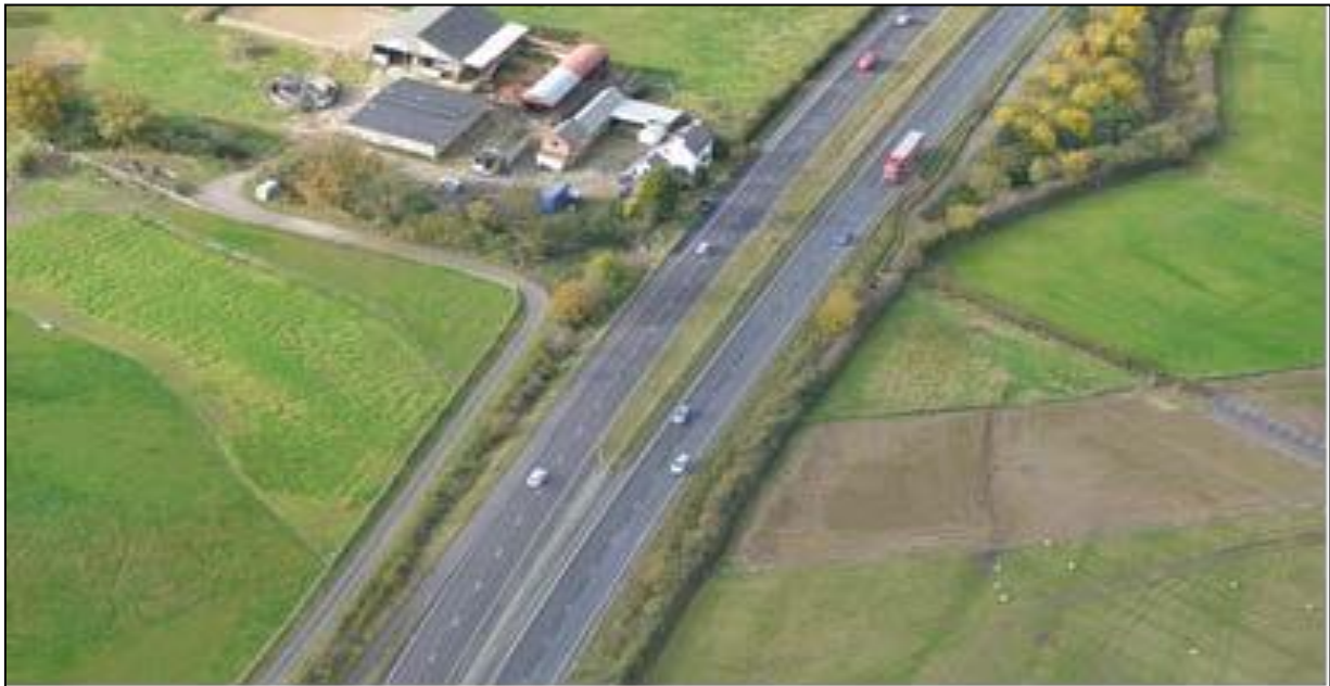
Figure 29: Cable corridor during restoration (courtesy of RWE renewables UK Ltd).
