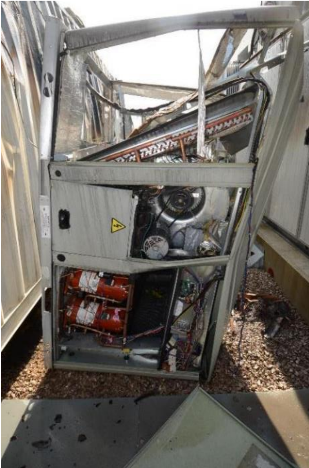
HVACS after coming dismantled from the container roof
