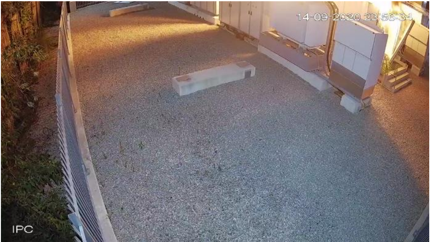
External CCTV showing the door being blown open and the smaller door coming detached
