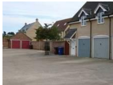
Photo of rear court
