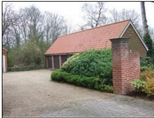
Example of well landscaped and designed garage (St. Mary's Court, Ipswich)
