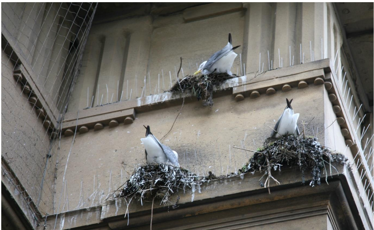
Photo 3.2.4. Kittiwake nests constructed on top of anti-bird spikes on the Guildhall at Newcastle Quayside
