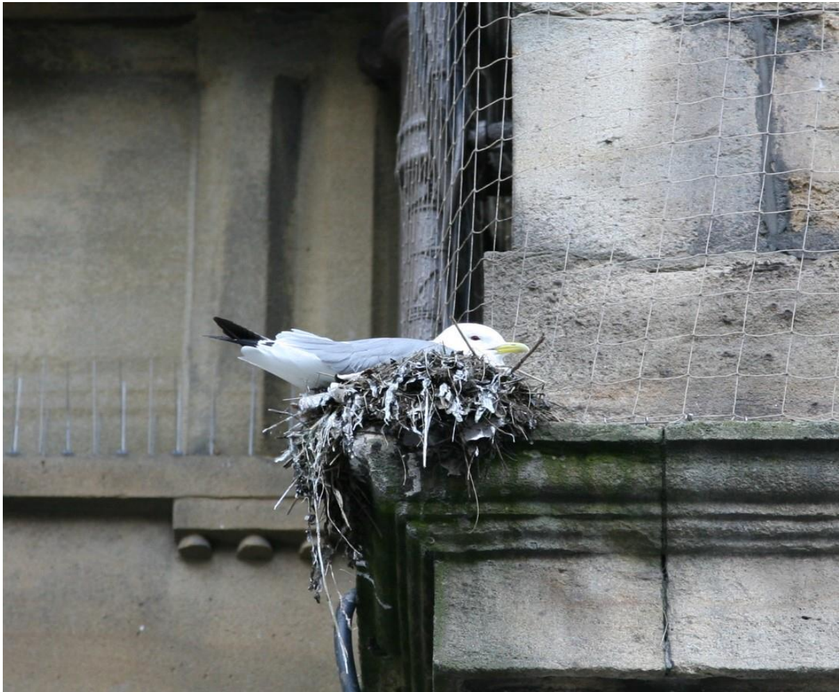
Photo 3.2.2. Kittiwake incubating on a nest constructed on top of exclusion netting on the Guildhall, Newcastle Quayside.
