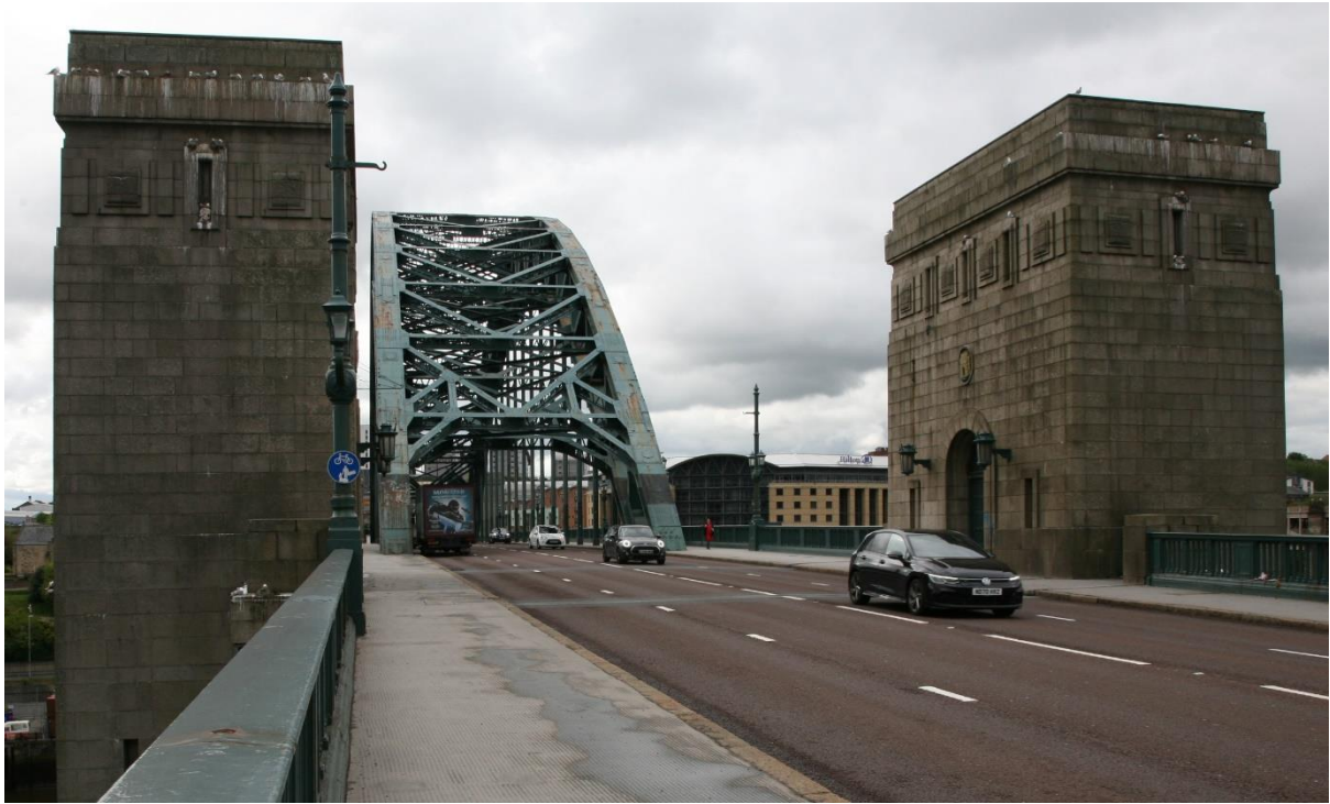
Photo D.16.5. Kittiwakes nest on the abutments above the road, close to passing heavy traffic, as well as on levels below the road; May 2021.
