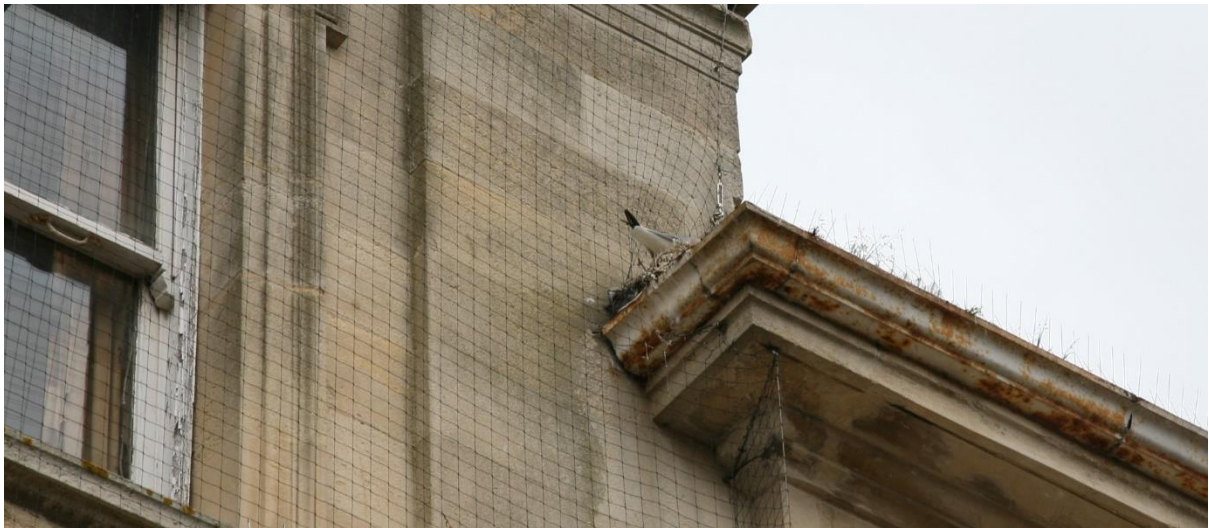
Photo E.17.6. 60 London Road North; May 2021.
