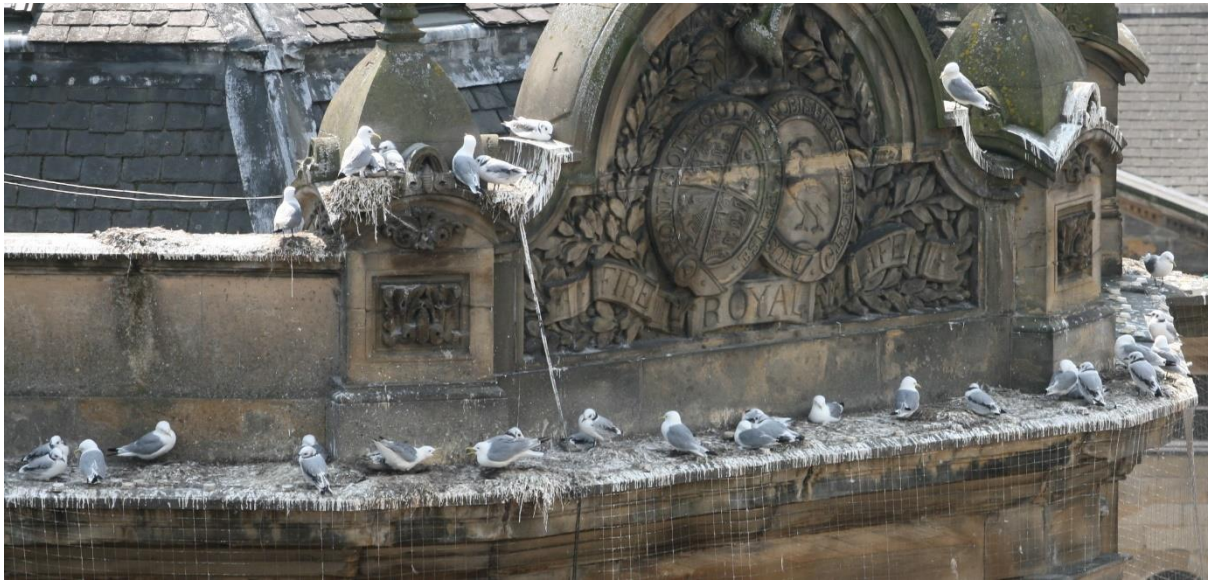
Photo D.7.2. Phoenix House (photographed from Tyne Bridge) showing an unusually wide ledge being used by kittiwakes and exclusion netting attached to that ledge with kittiwake nests built on top of the netting; July 2021.
