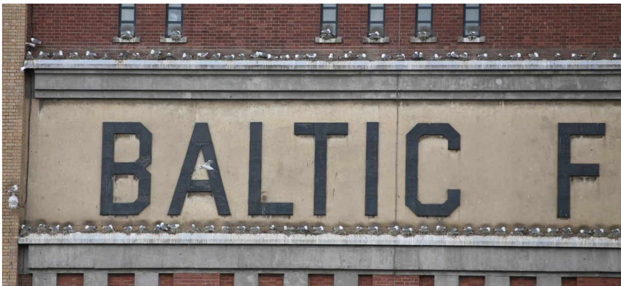
Photo D.4.2. Part of north face of Baltic Flour Mill; May 2021.
