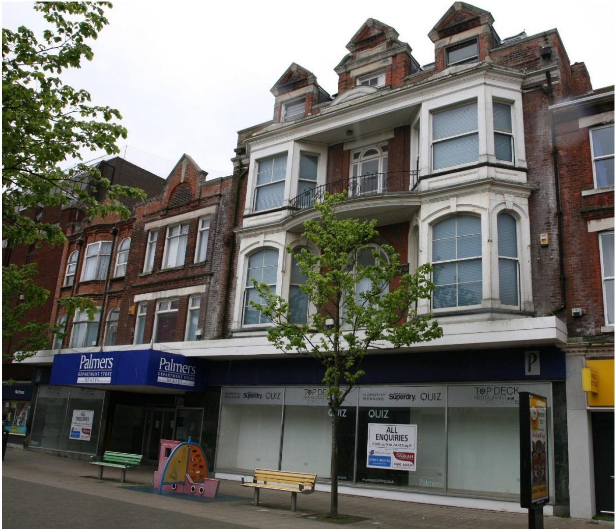
Photo E.17.4. Number 59 London Road North; May 2021.
