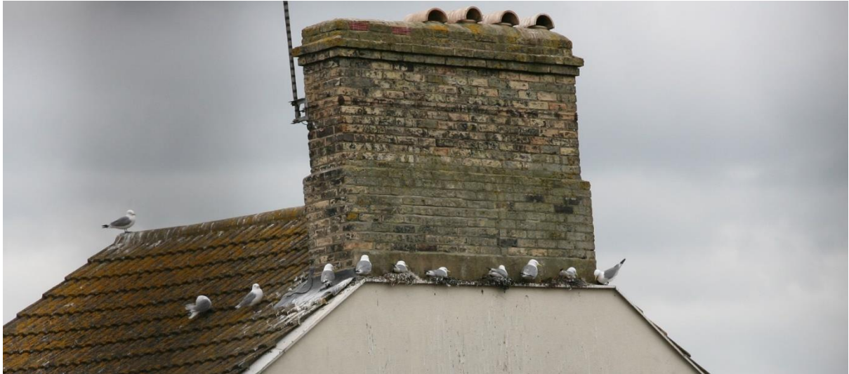
Photo E.15.1. Kittiwake nests on the end wall of 13 Clapham Road South, across the road from the BT building; May 2021.
