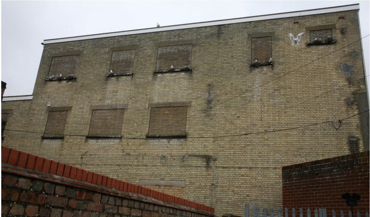
Photo E.20.1. This warehouse site on Gordon Road was overlooked in May and so not included in the study of nest site features and breeding success; Photo June 2021.
