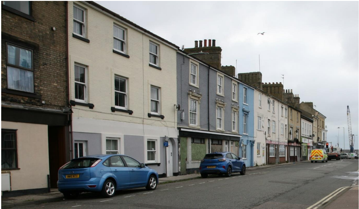
Photo E.5.1. Properties in Commercial Road; May 2021.
