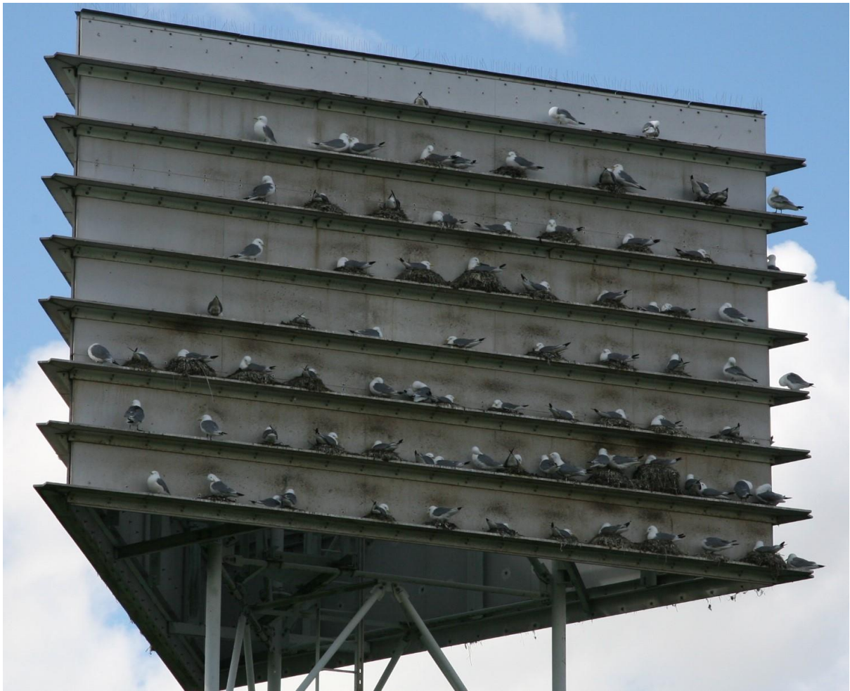
Photo D.3.4. East face of Saltmeadows tower, Gateshead; May 2021.
