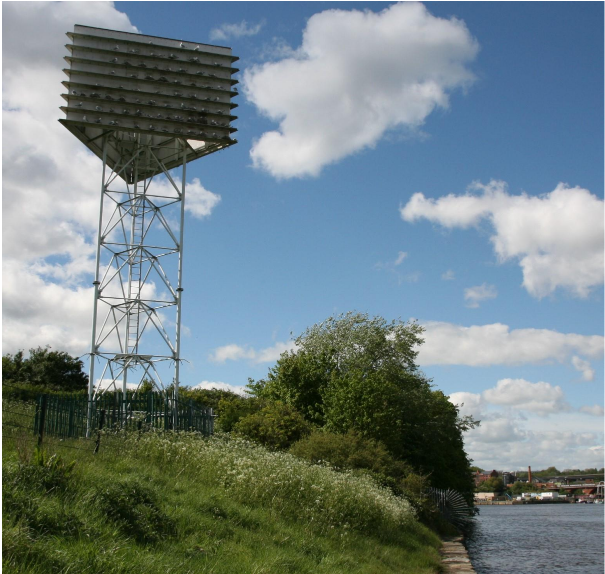
Photo D.3.2. Saltmeadows tower, Gateshead, photographed from the south-east, showing its lean off vertical that increases solar exposure for nests on the South-West face and reduces exposure for nests on the East face; May 2021.
