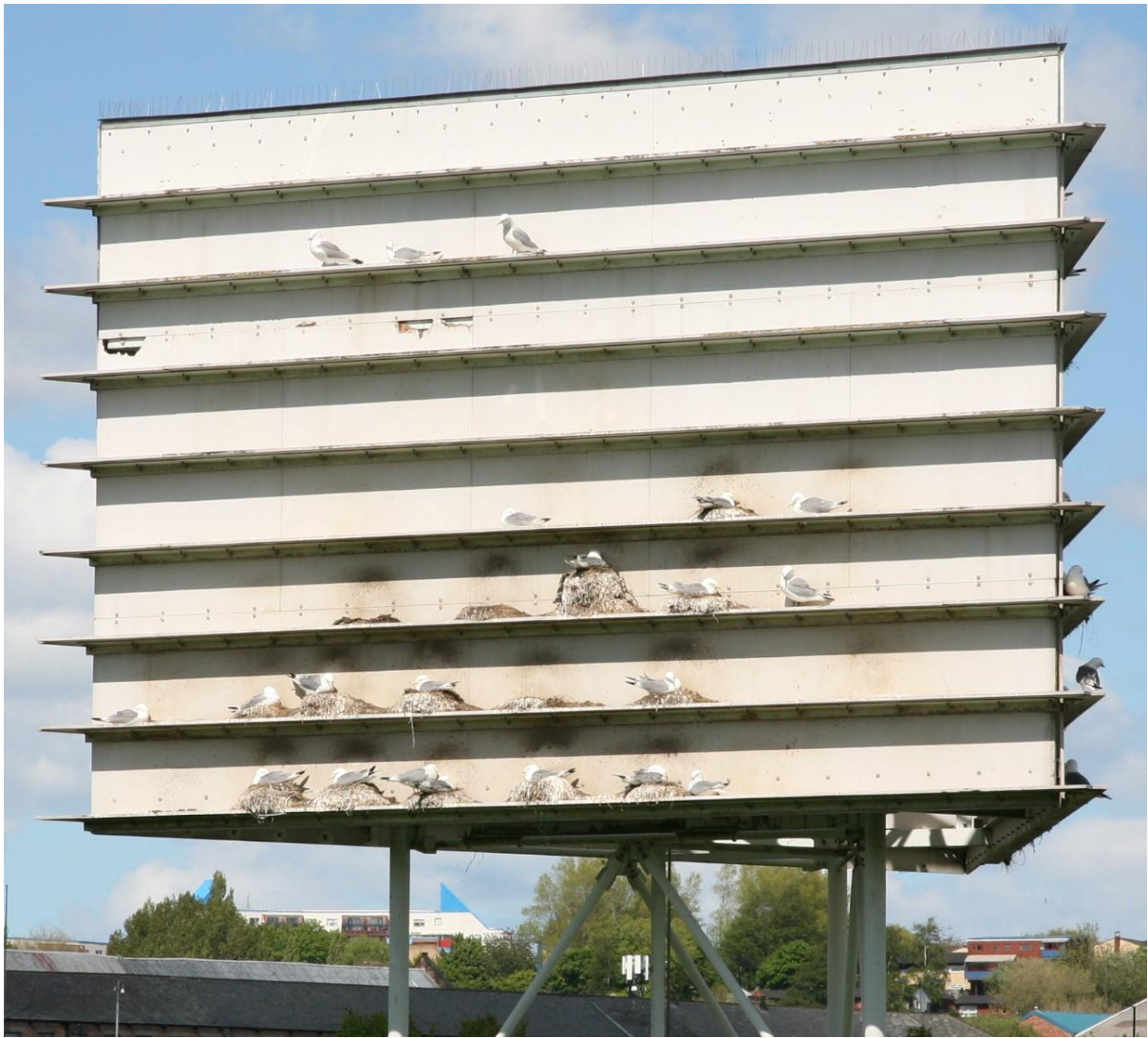
Photo D.3.3. South-West face of Saltmeadows tower, Gateshead; May 2021.
