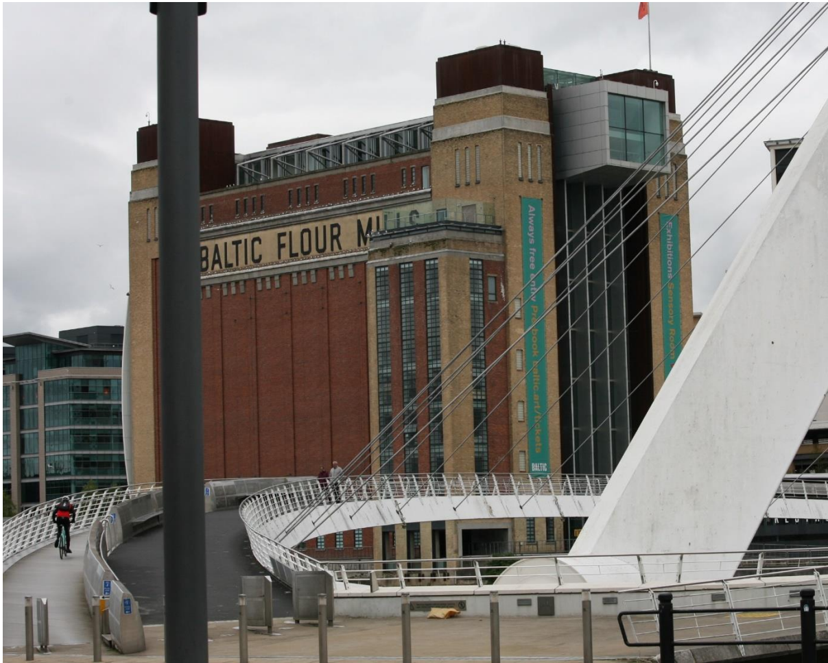
Photo D.4.1. Baltic Flour Mill (Baltic Arts Centre, Gateshead), from the Newcastle Quayside of the river looking across the Millennium Bridge. Kittiwakes nest mainly on the two long ledges above and below the name; May 2021.
