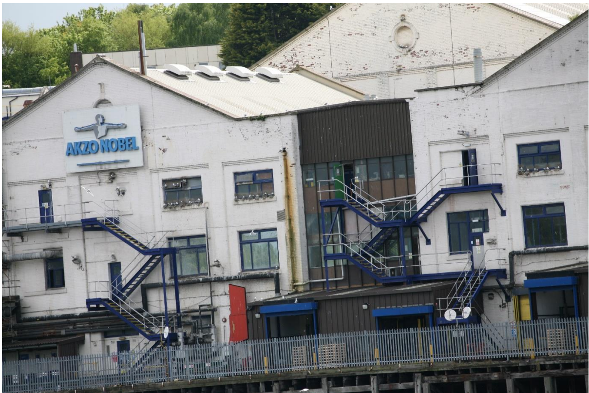
Photo D.2.2. Akzo Nobel, showing kittiwake nests on window ledges on the north-facing side of the industrial buildings on the south bank of the River Tyne; May 2021.
