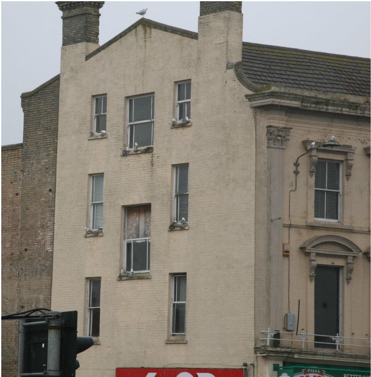
Photo E.6.4. The Station Square building above Papa John's, where the upper part of the building front has had exclusion netting fitted early in 2021. Kittiwakes now nest on window ledges on the end of the building that had not previously been occupied; June 2021.
