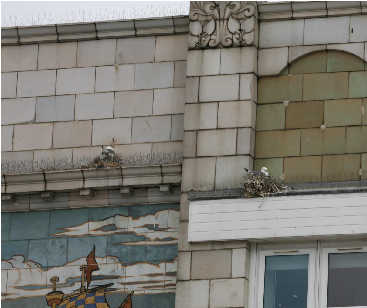
Photo E.7.1. Kittiwakes nesting on the Columbus Building, despite presence of anti-bird spikes along the ledges; May 2021. These nests overlook the busy A47 trunk road through Lowestoft, and immediately across the road is the major construction work for the enhanced flood defences.
