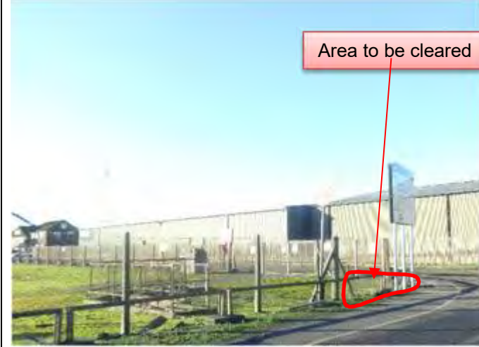
8.4.2.3. – View at crossing
