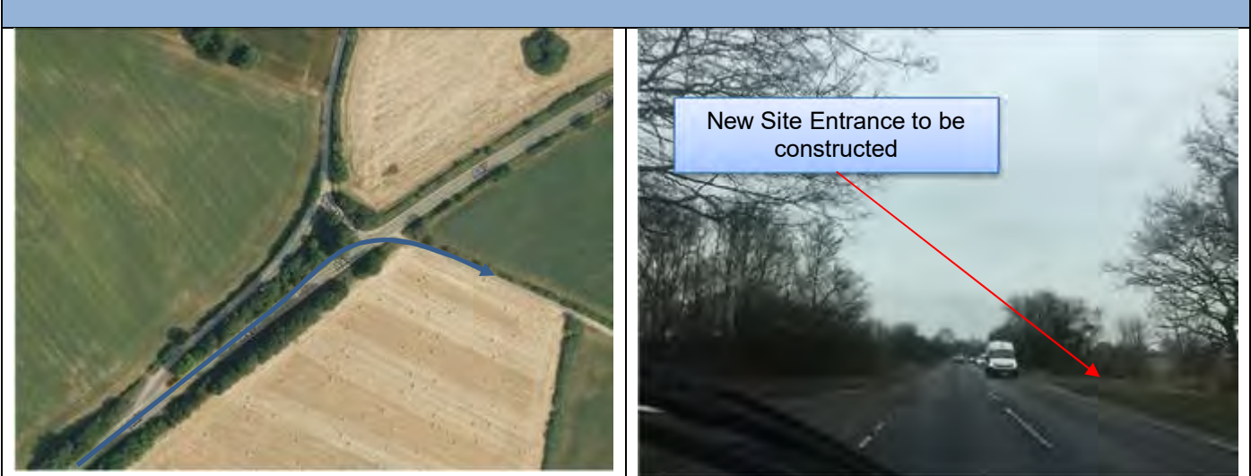
8.8.5.1. – Aerial View of Location 8.8.5.2. – View of entrance to roundabout
