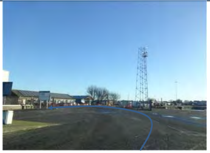
8.4.1.2. – View prior to junction
