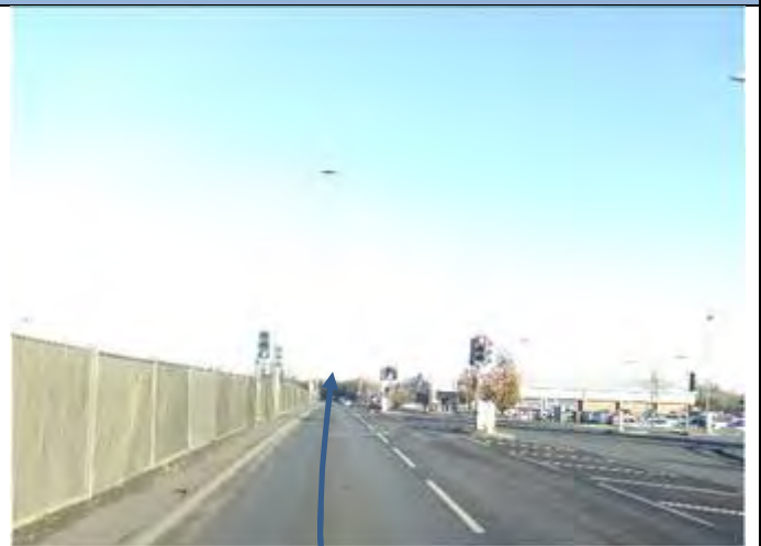
8.4.5.2. – View of splitter island
