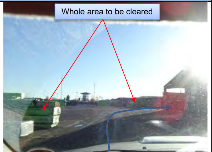
8.4.3.2. – View prior to bend
