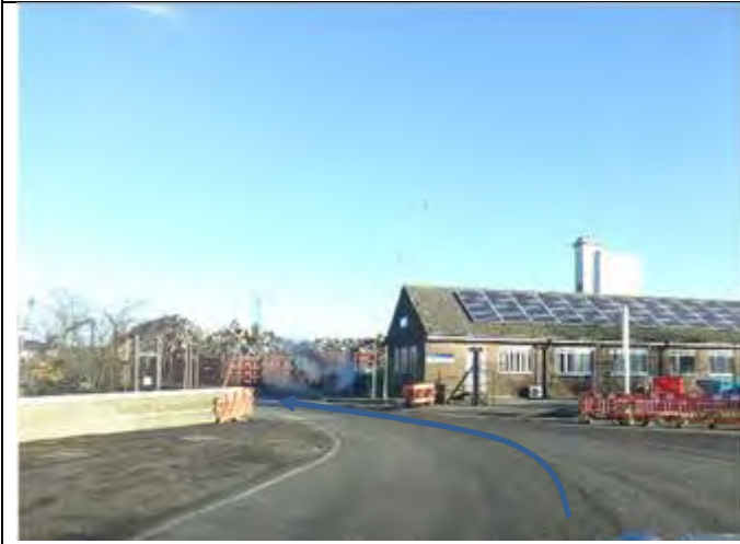
8.4.1.3. – View at crossing
