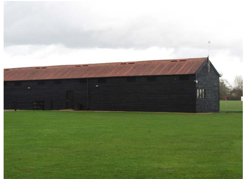
Figure 2. Barn vernacular with dark weatherboard cladding
