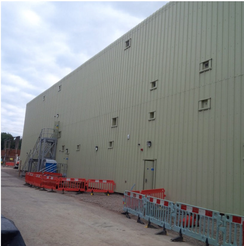
Figure 5. Gas insulated Substation building clad in metal sheet
