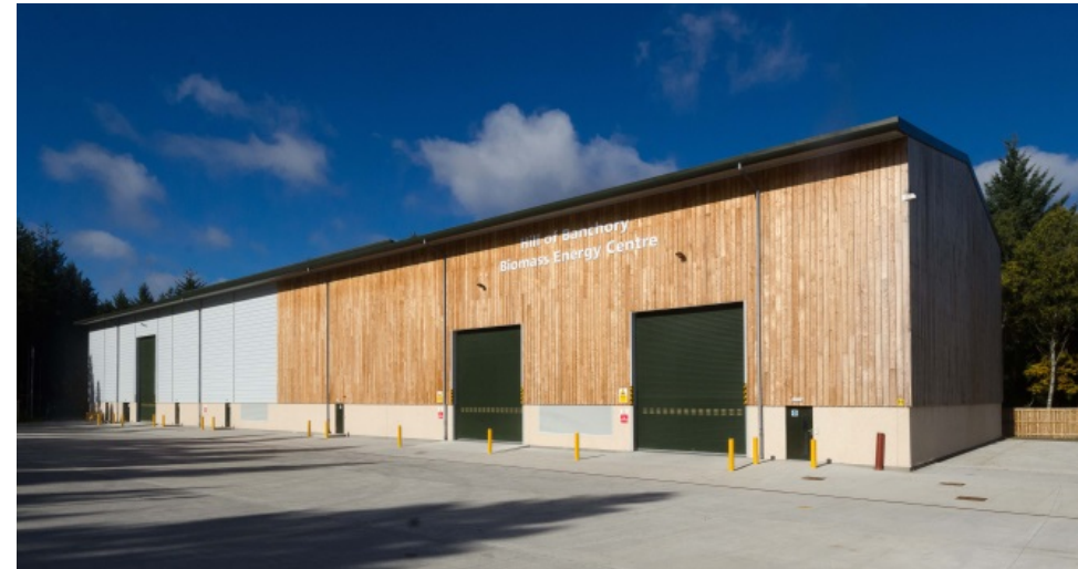
Figure 4. Biomass centre with wooden cladding
