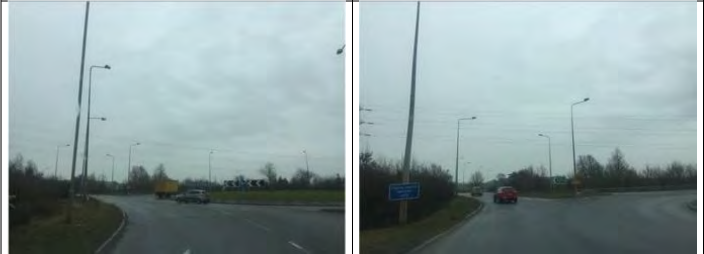
8.7.3.3. – View on roundabout 8.7.3.4. – View of exit of roundabout
