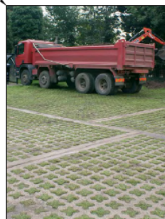
TYPICAL GRASSCRETE PAVING AFTER INSTALLATION
