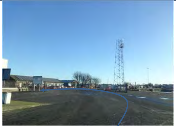
8.4.1.2. – View prior to junction
