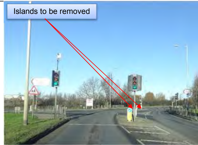
8.4.6.3. – View on junction
