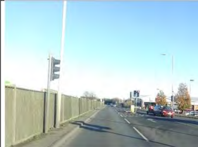
8.4.5.3. – View on junction
