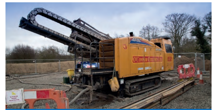
Example Horizontal Directional Drilling (HDD) Rig
