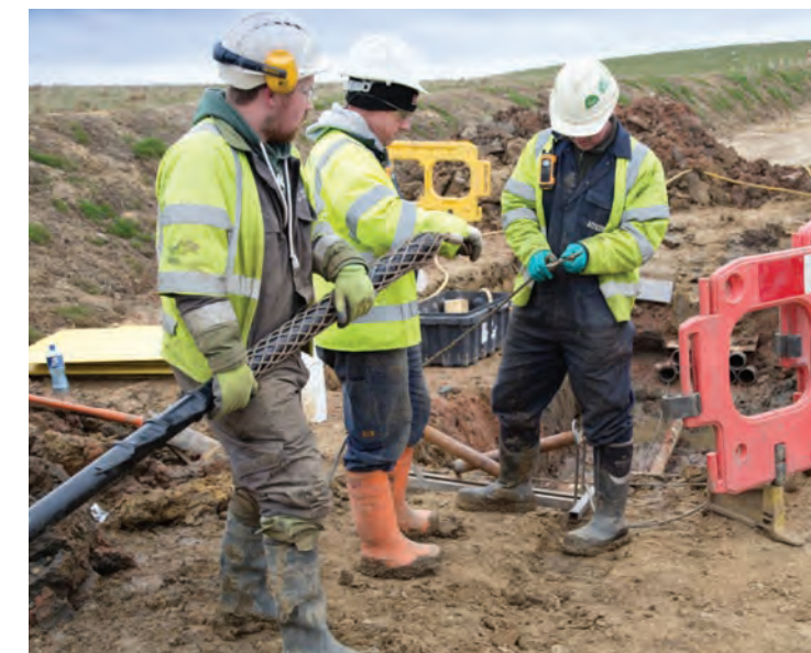
Cable pulling preparation
