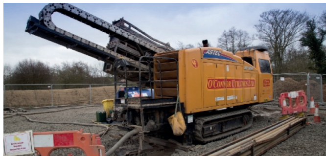
HDD unit, showing the drill rig and drilling pipes.
