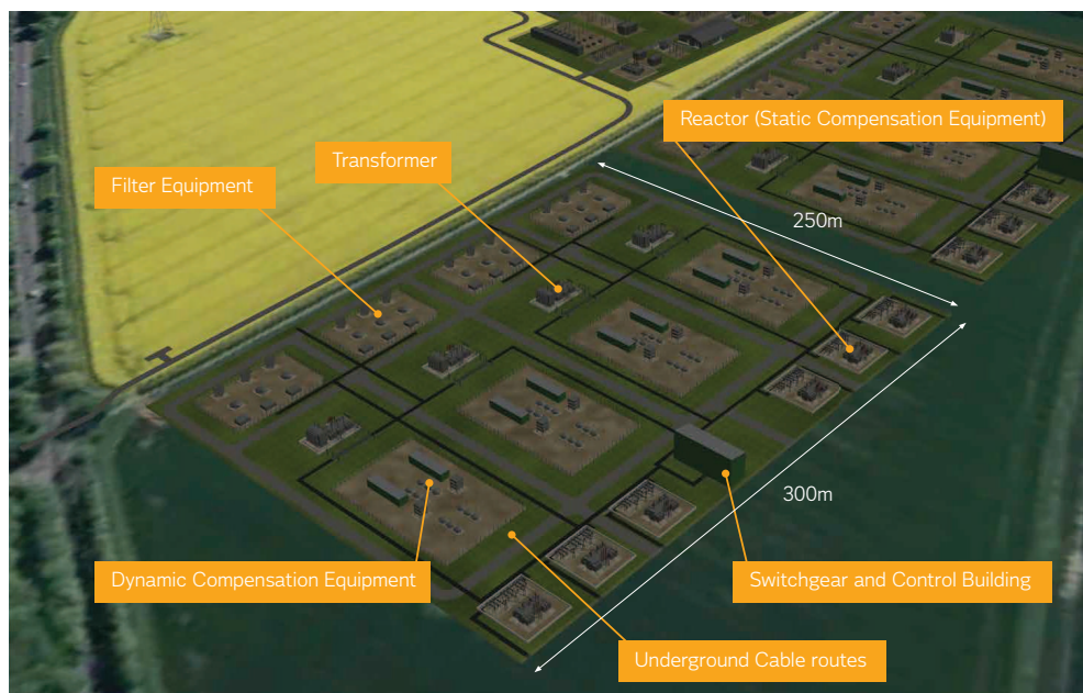
3D visualisation of project substation (HVAC option)
