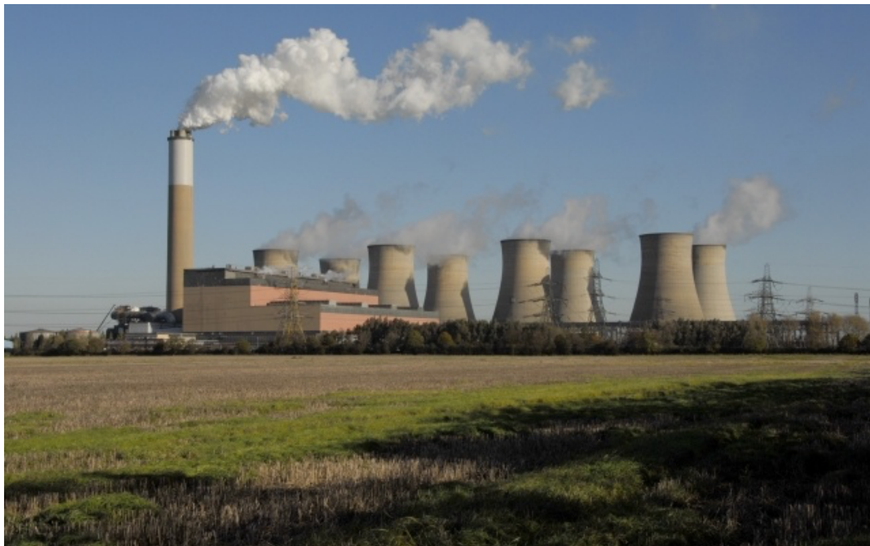
Cottam power station
