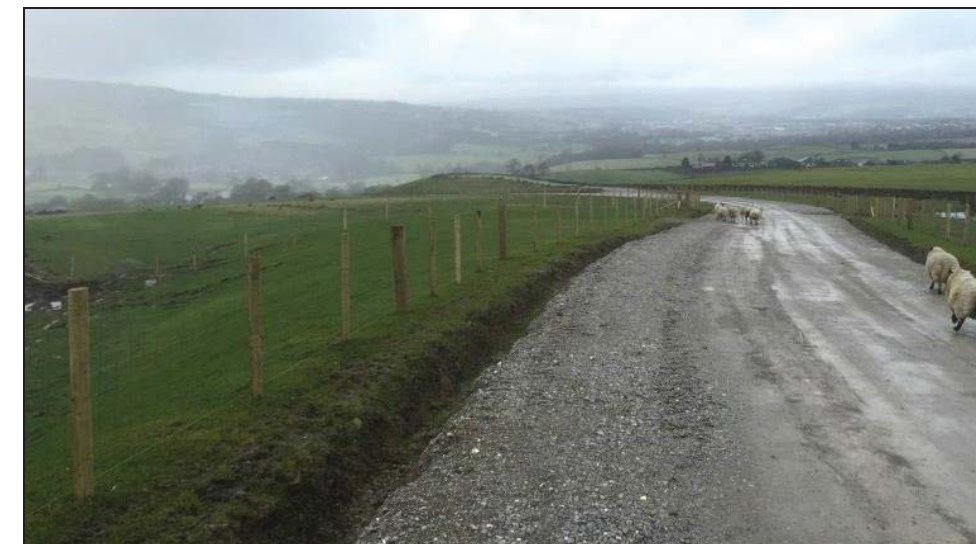
Plate 6: Typical drainage ditch adjacent to access track
