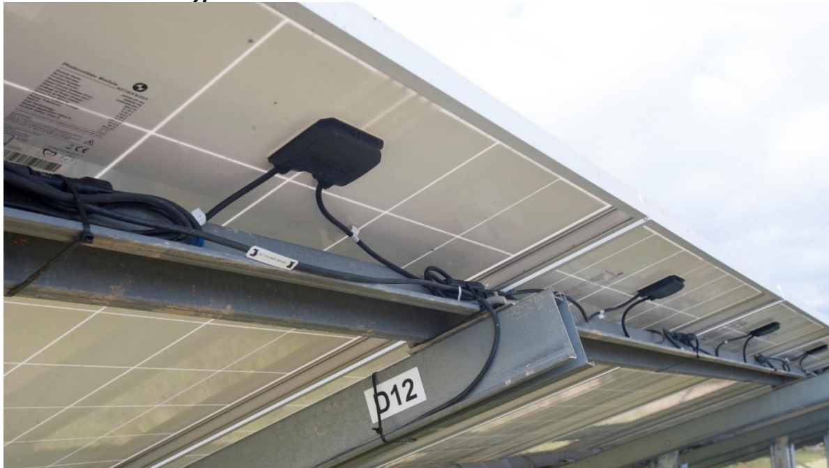
Plate 5.5c Typical underside of solar PV modules
