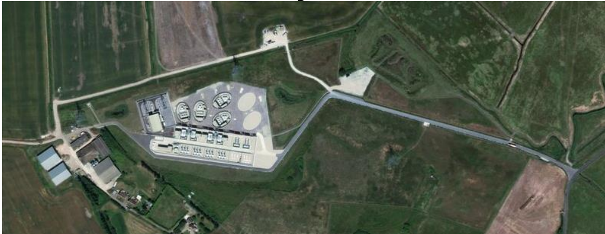
Plate 5.4 Aerial Photo of the existing Cleve Hill Substation 1
