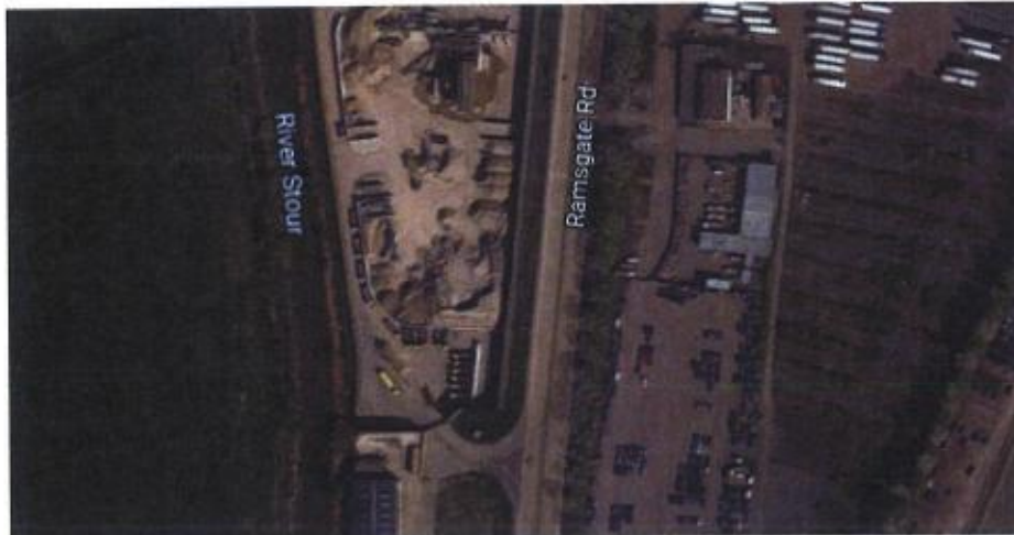
Figure 8 – Ramsgate Road Accesses
