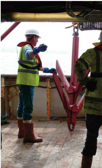
Activities such as pre-lay grapnel runs have a high chance of encountering archaeological materials.
