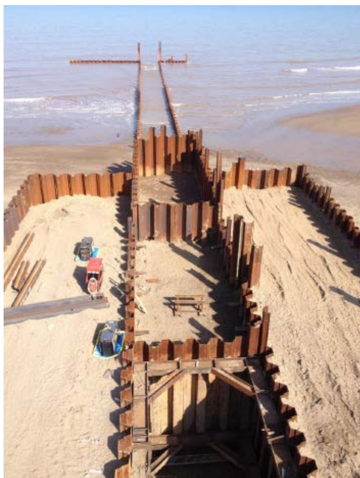
Figure 2-6: Illustration of sheet piling used for intertidal cofferdams (Sheet Piling UK Ltd).
