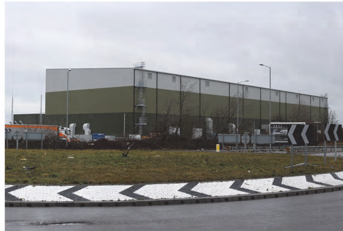
R - Nemo Substation from Richborough Roundabout
