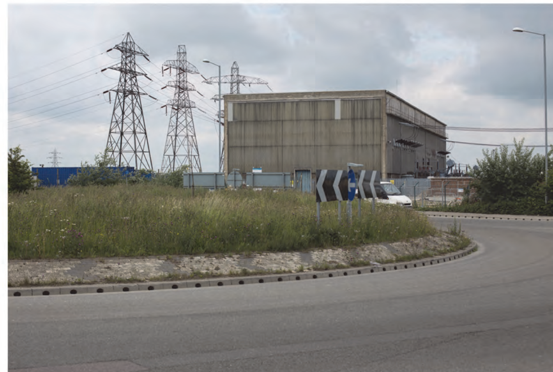
T - Existing Thanet Wind Farm Substation
